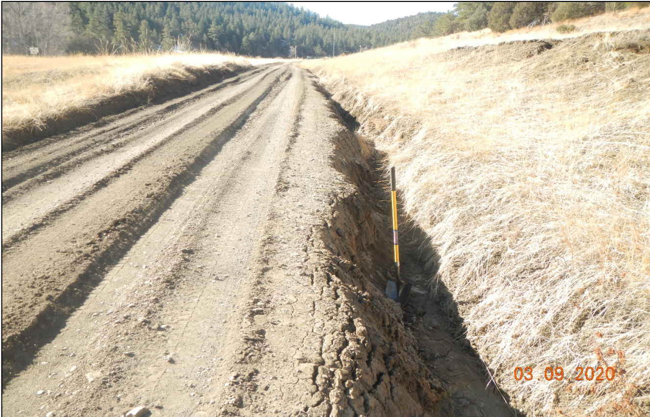
Photo 4. The sides of the main road has eroded a deep channel at Lat/Long:37.041830,-104.81016.
