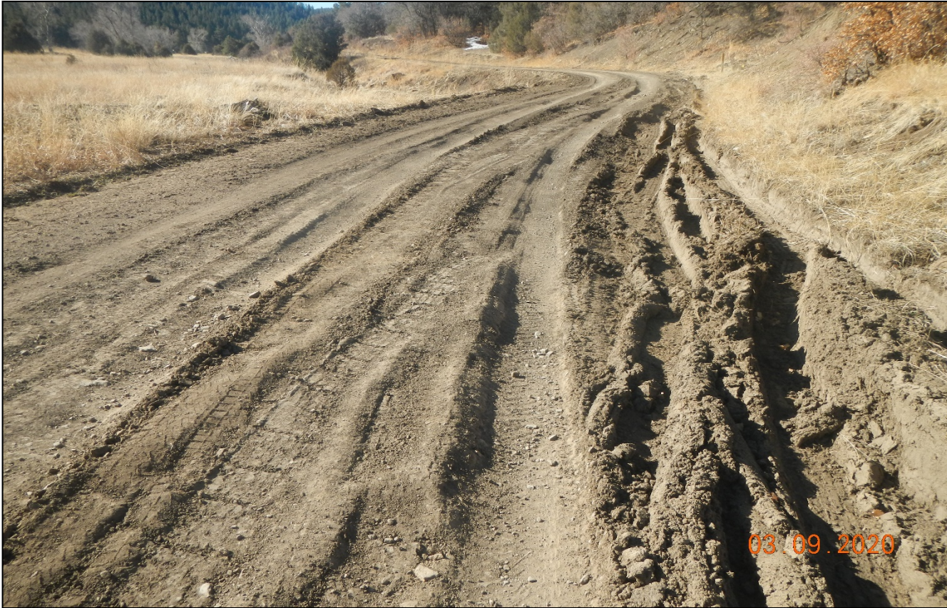
Photo 3. There is vehicle rutting along the main access road near the location.
