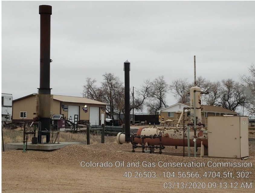
Photo #3 Separator & ECD
