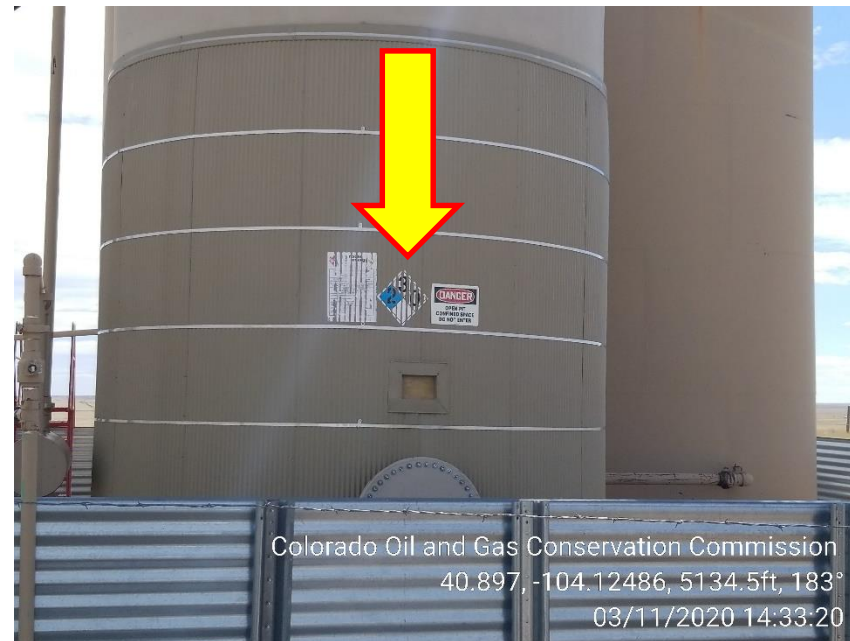
Photo 4 – Produced Water Tank missing Capacity and NFPA Label is fading.
