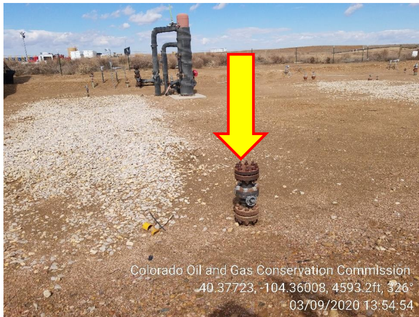
Photo 7 – Unmarked Risers at Compressor
