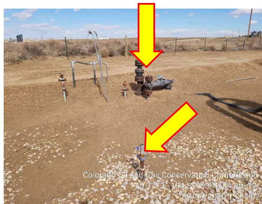
Photo 4 – Unmarked Risers at Compressor
