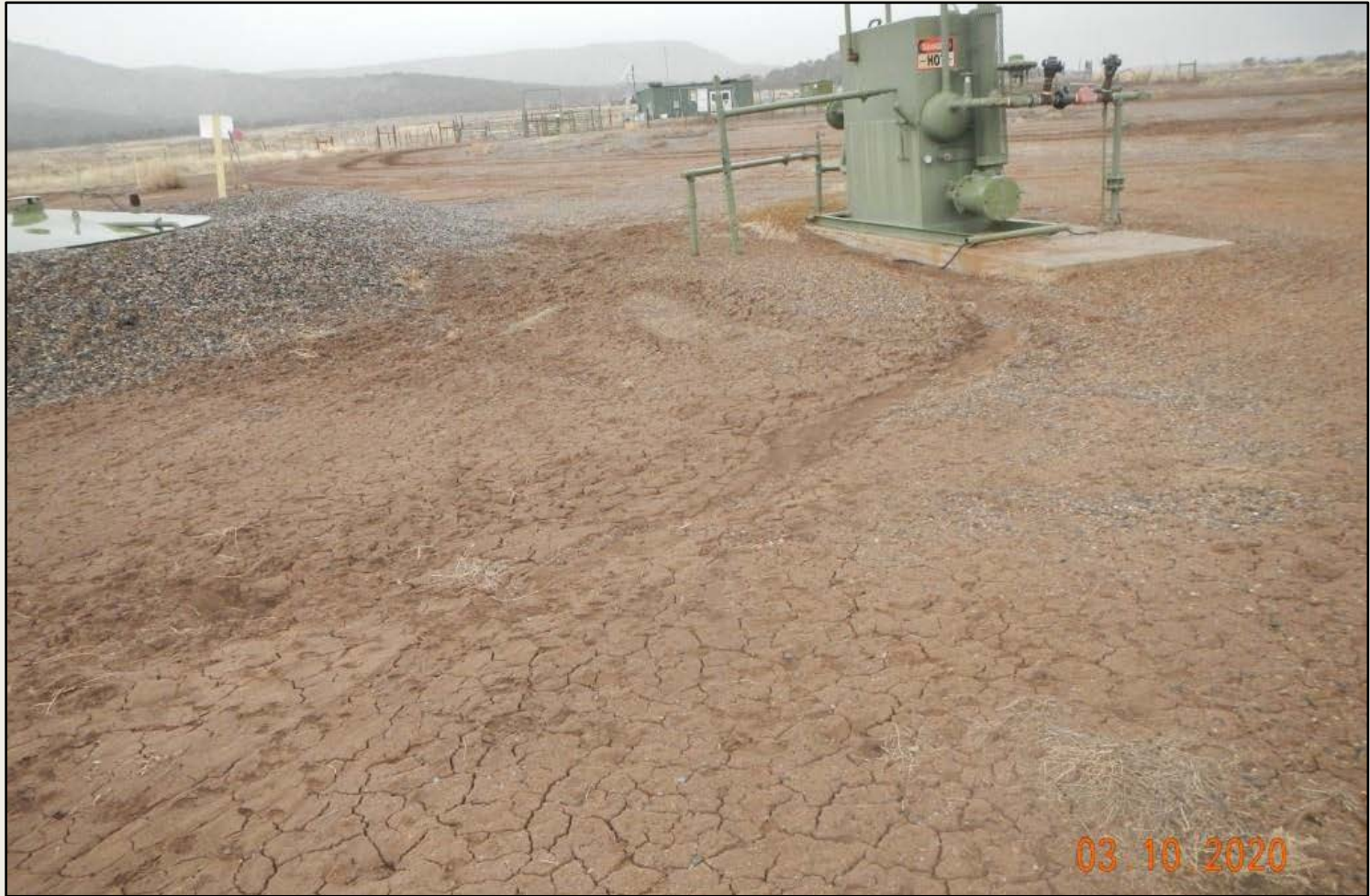
Photo 3. View of area where stormwater flows around facilities creating erosive channel.
