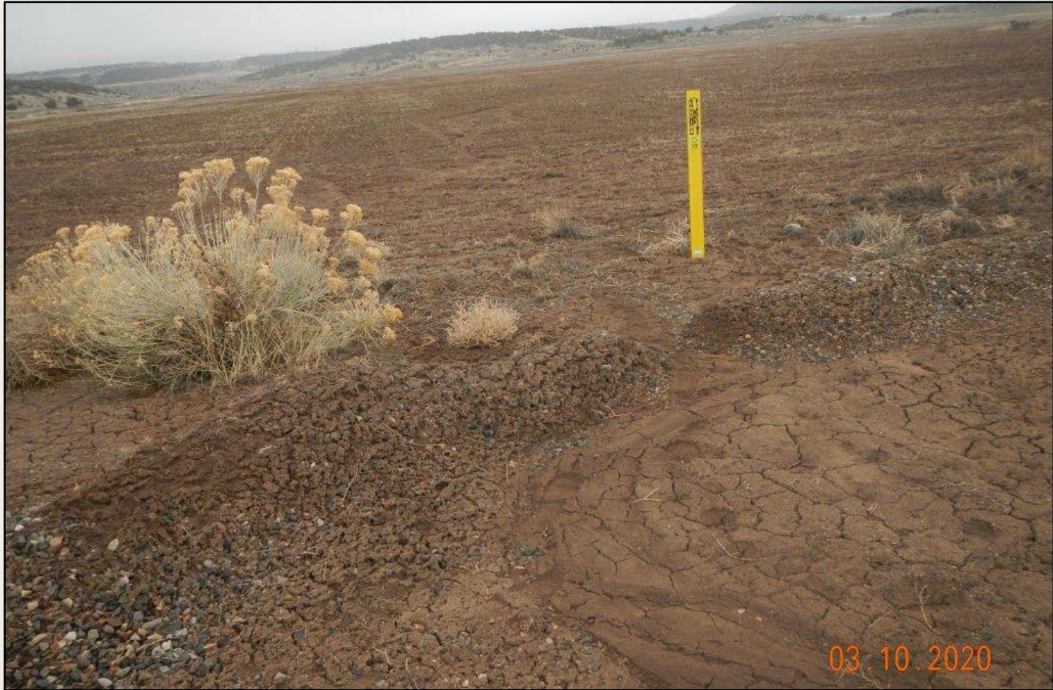
Photo 2. View of erosional channeling and failed berm within the southeastern project area.
