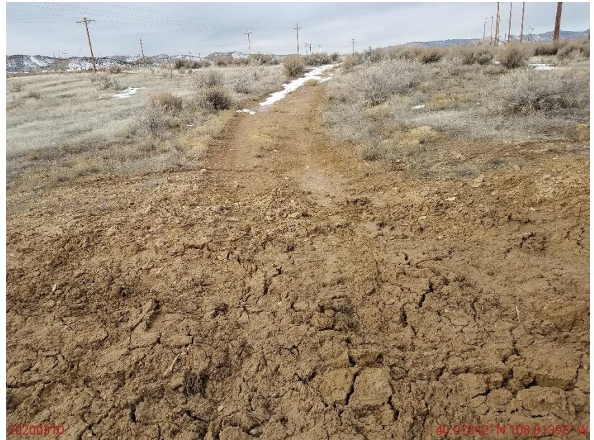
Photo 10: Photo taken from the west end of the Location, facing west. Photo shows access road has not been reclaimed per corrective actions.
