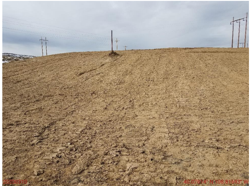
Photo 6: Photo taken from the east end of the Location, facing west. Photo shows Operator installed tracking on the slopes of the reclamation areas; Tracking is a temporary control and will not be sufficient for long term stabilization until vegetation has established. Tracking should also be used in conjunction with other BMPs per good engineering practices.
