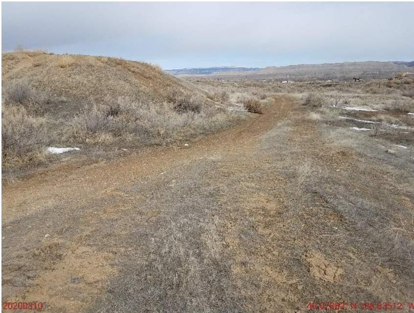
Photo 9: Photo taken from the north end of the Location, facing north. Photo shows access road has not been reclaimed per corrective actions.
