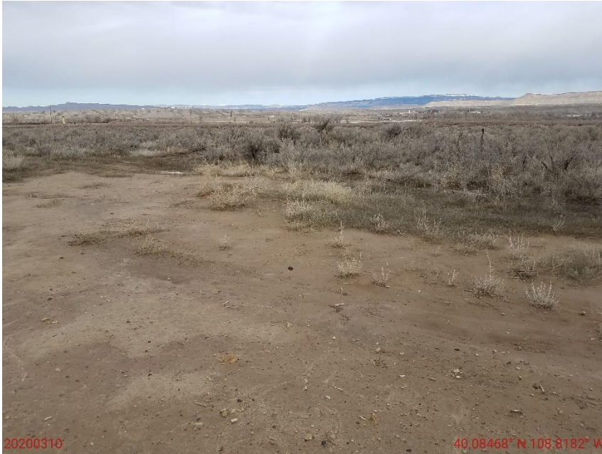
Photo 1: Photo taken from the south end of the Location, facing north. Photo shows Location; A pipeline has been constructed on the south end of the Location.
