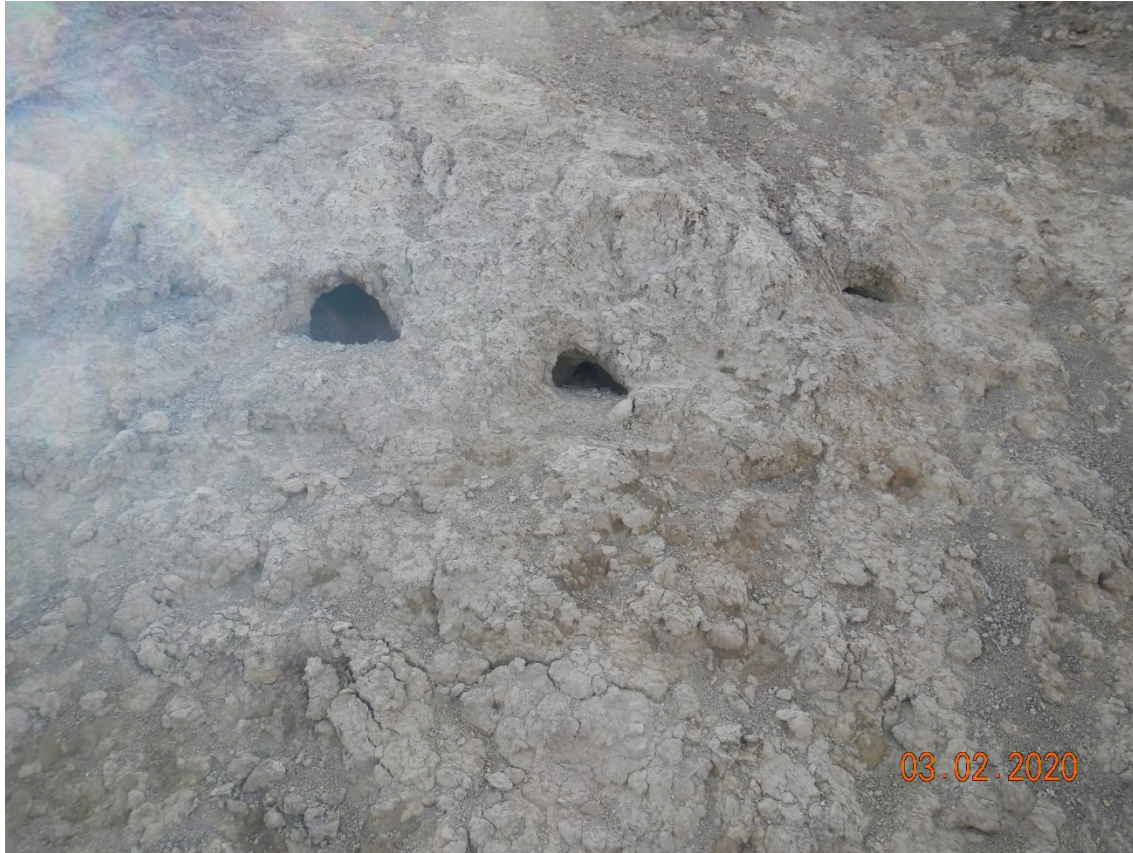
Photo # 24 – Produced water pit east berm animal burrows
