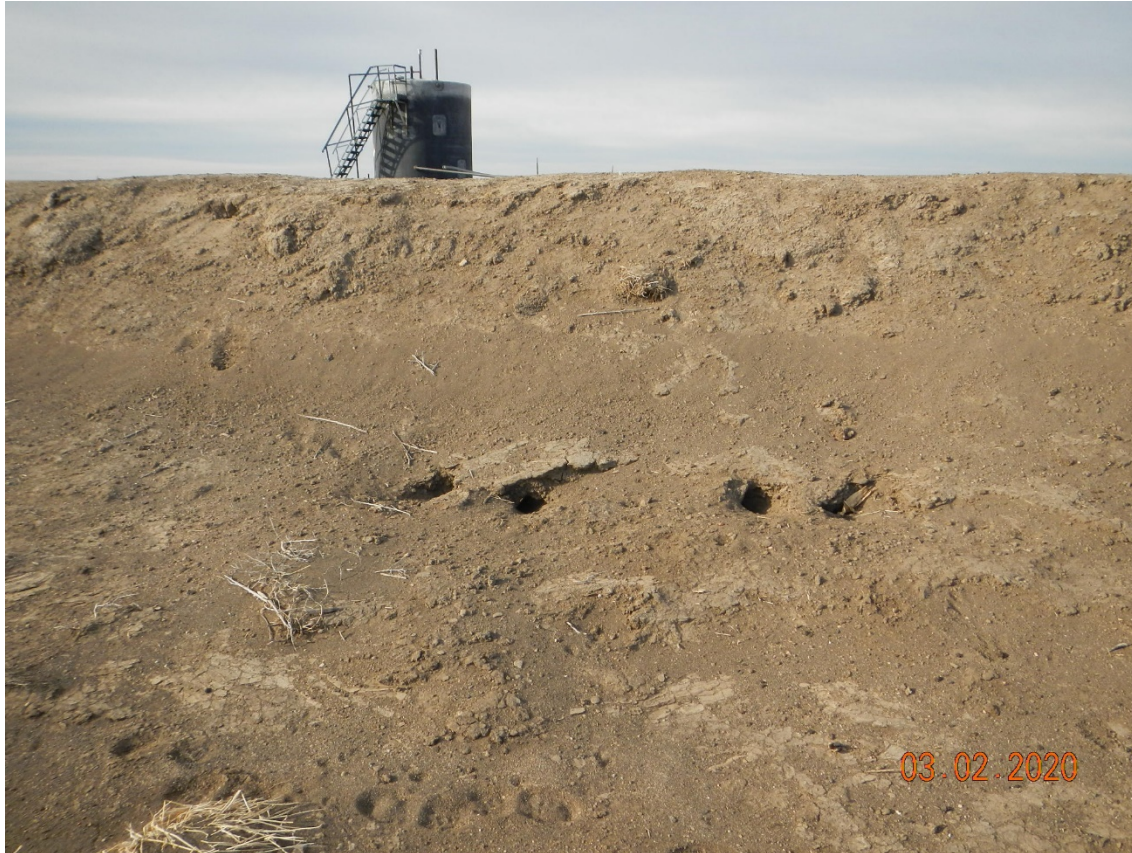
Photo # 26 – Produced water pit south berm animal burrow
