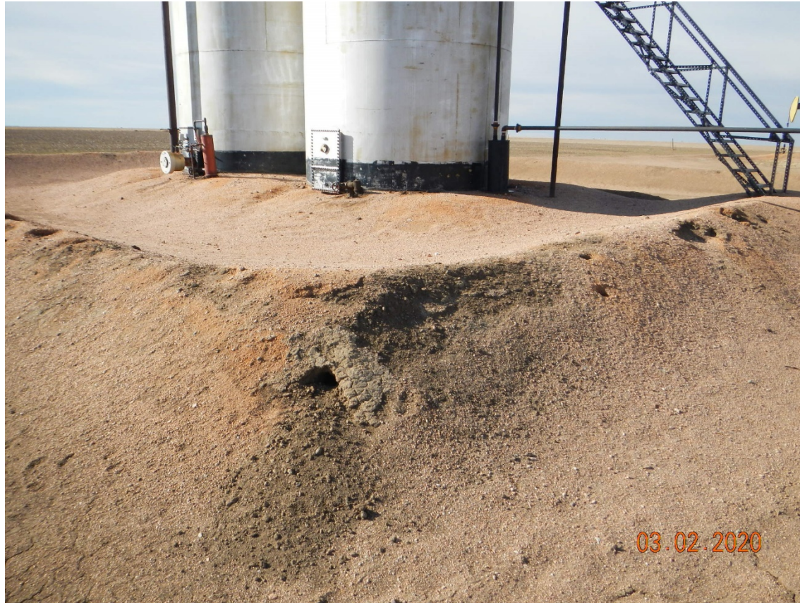
Photo # 3 – Crude oil tank battery southeast corner view northwest. Animal burrows in the berm
