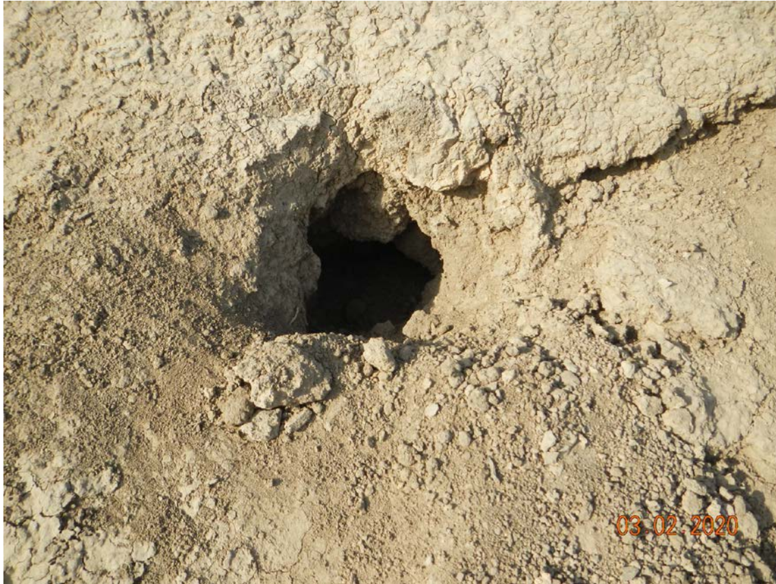
Photo # 25 – Produced water pit south berm animal burrow
