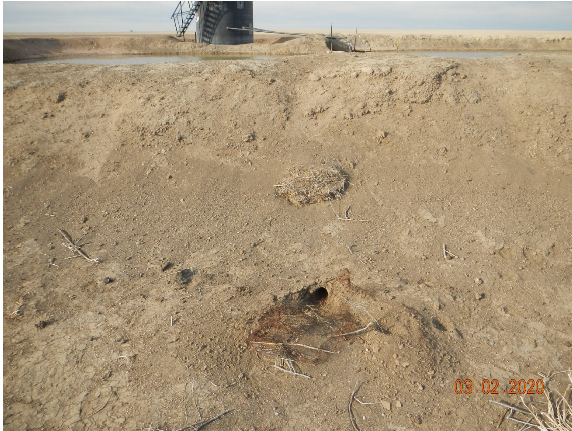
Photo # 27 – Produced water pit south berm animal burrow
