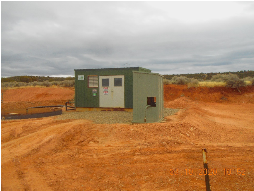
Pump housing. Meter shed.
