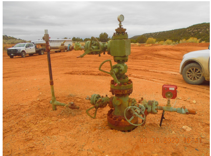
Injection wellhead..
