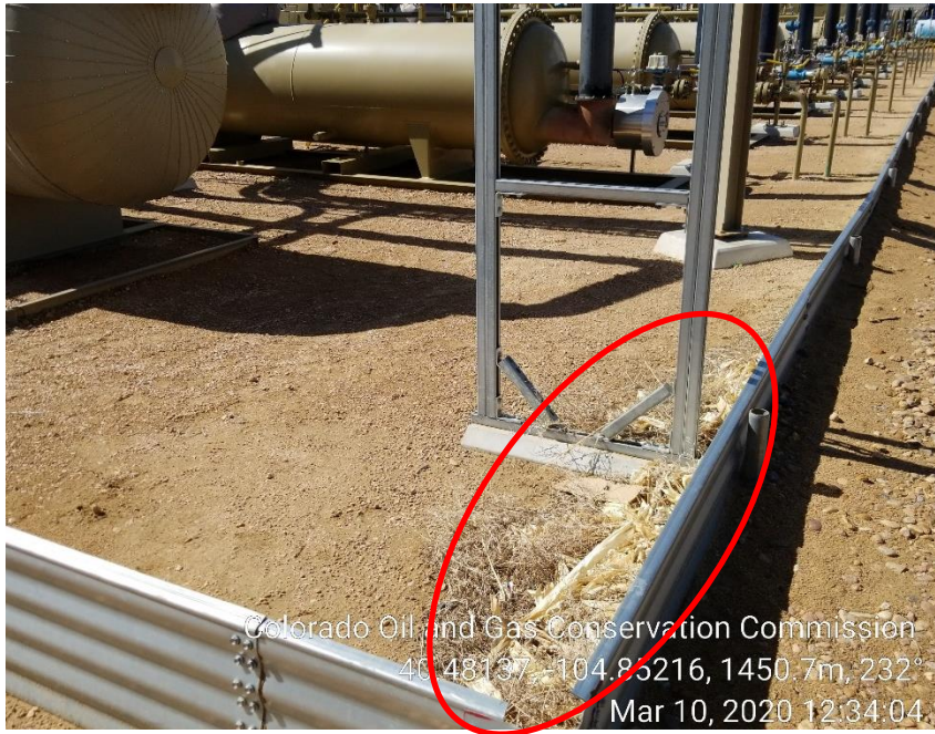
Photo 23: Debris in separator berm (north east corner)
