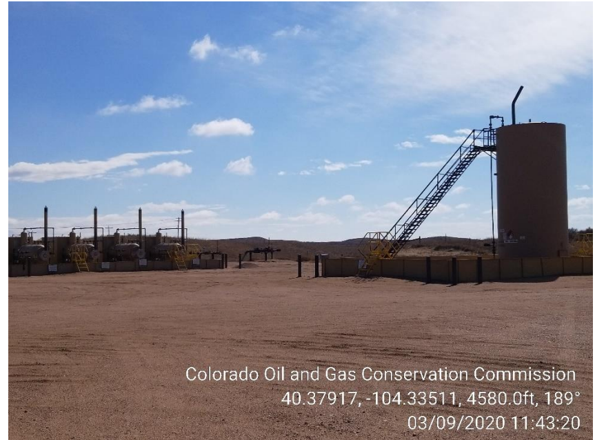
Photo 2 – Tank Battery
