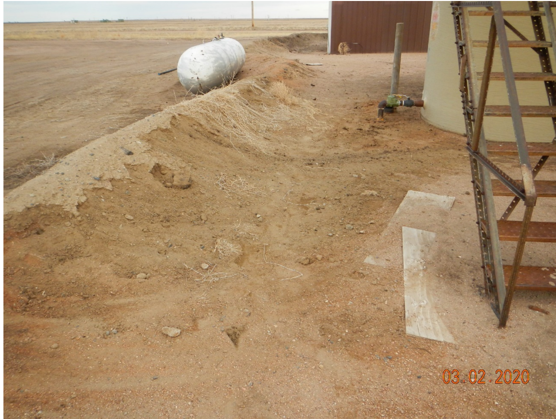
Photo # 10 – Inner wall of containment berm, west side of injection shed, scraped significantly
