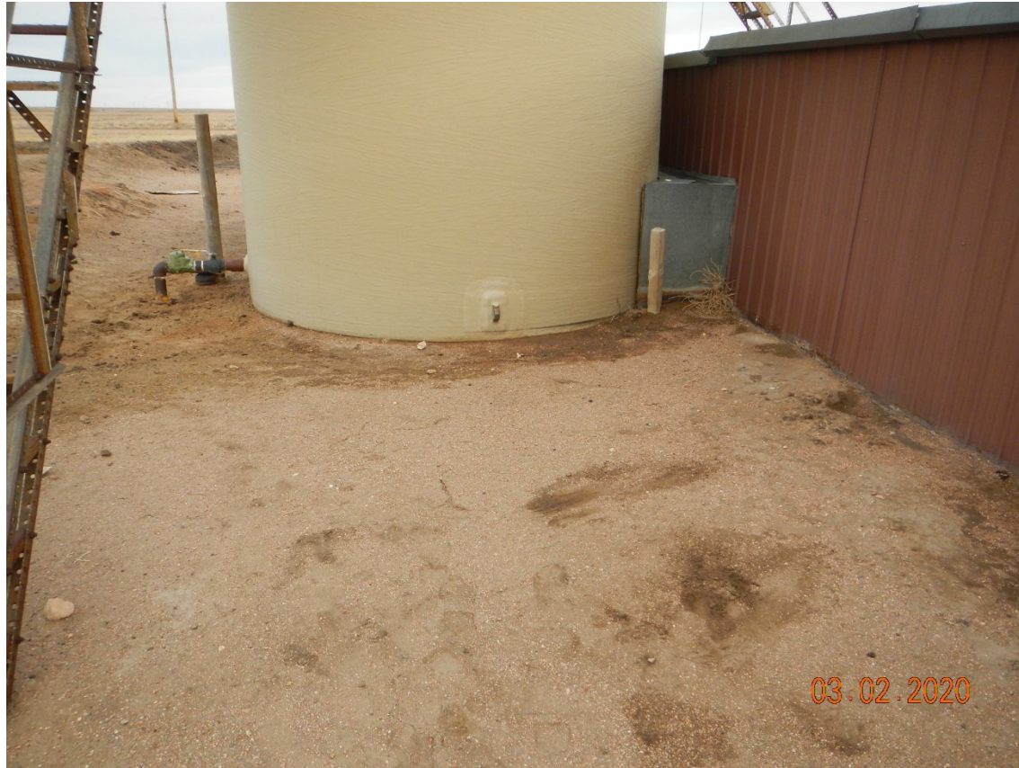
Photo # 6 – Wet area around base of produced water tank extending from injection shed to containment berm
