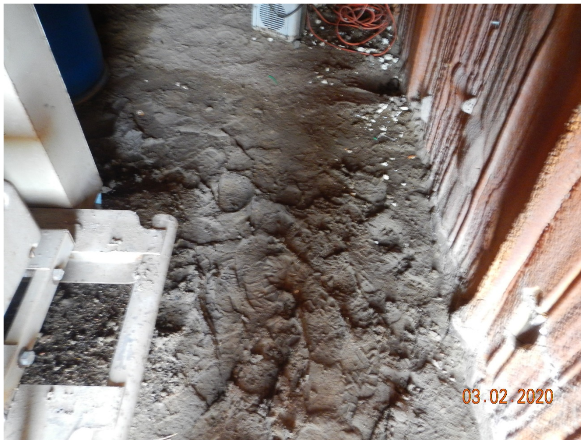
Photo # 3 – Head of shallow trench leading out from under injection house eastern wall at wet-dry line in soil
