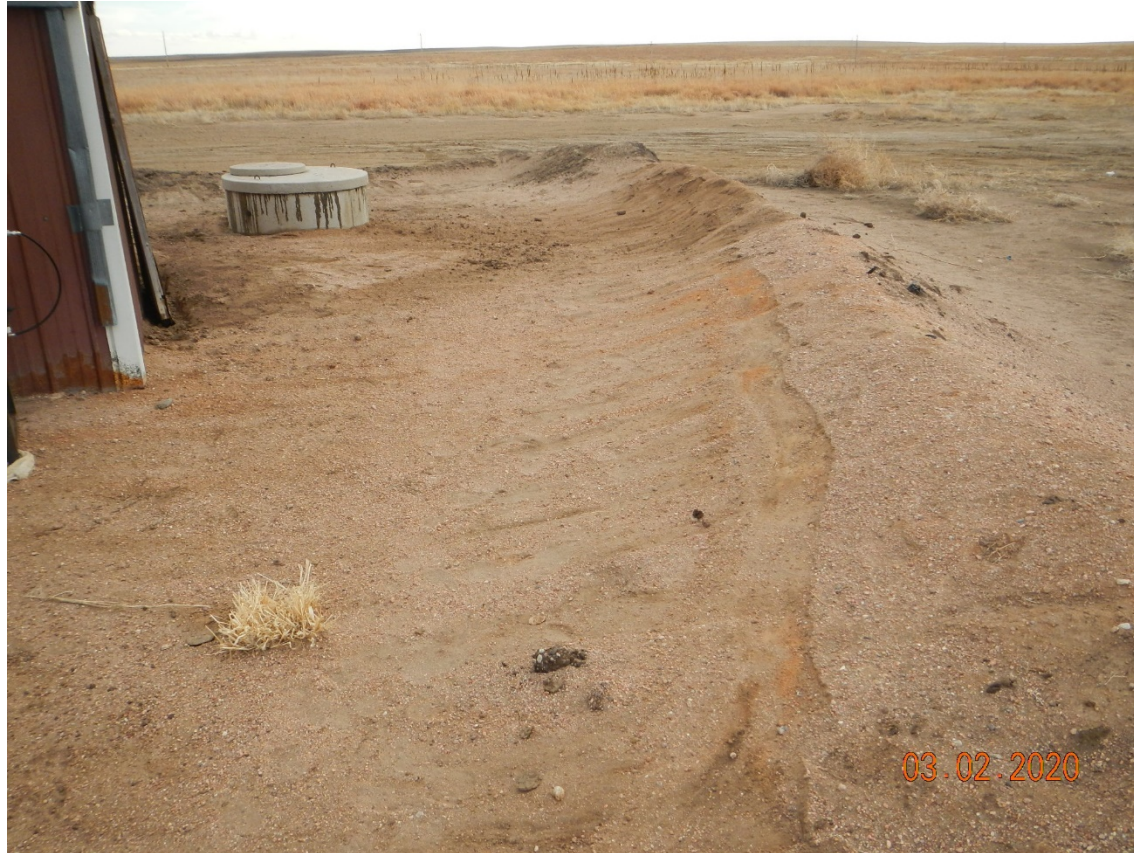
Photo # 11 – Inner wall of containment berm, west side of injection shed, scraped significantly
