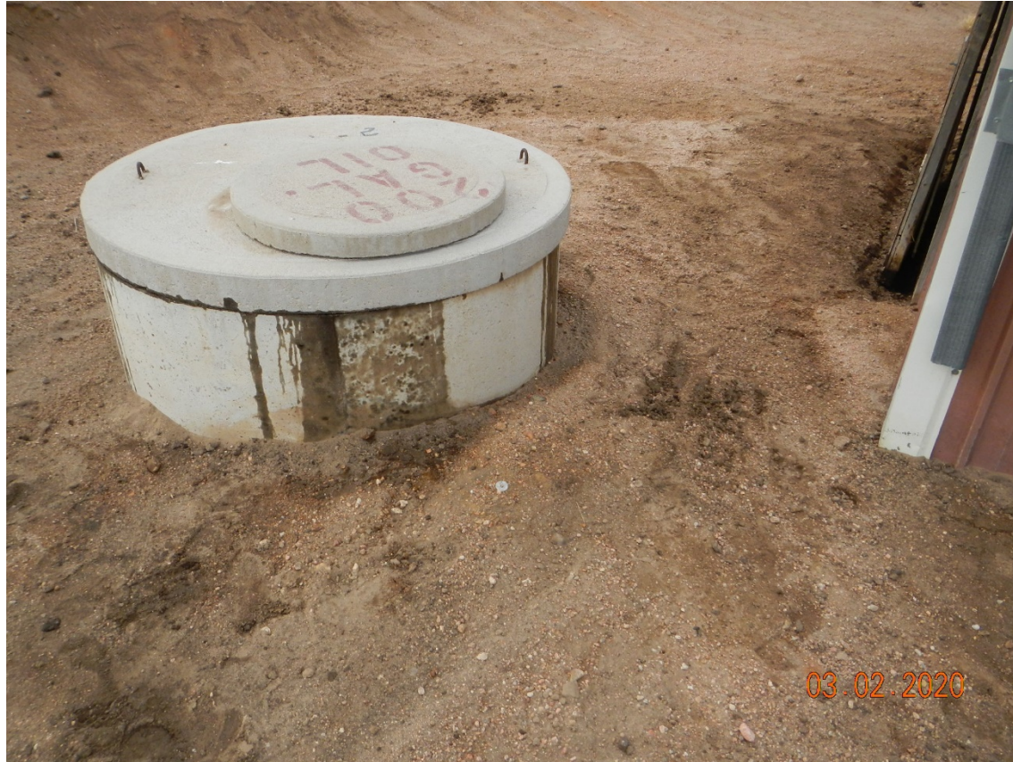
Photo # 7 – Wet area around base of concrete oil vault, staining on side of vault, appears to have overfilled
