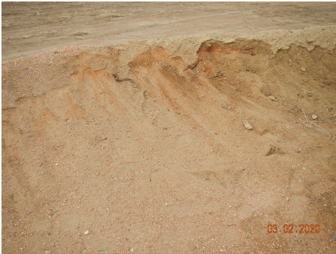
Photo # 9 – Inner wall of containment berm, west side of injection shed, scraped significantly
