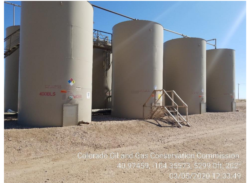
Photo 4 – Eastside Tanks – Content and Capacity is Fading
