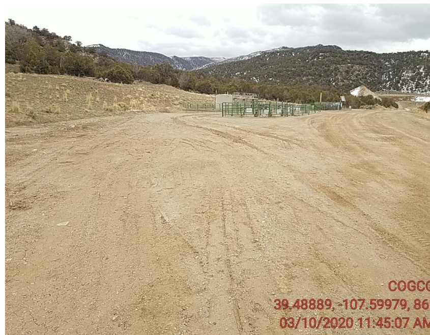
Frack tank is gone
