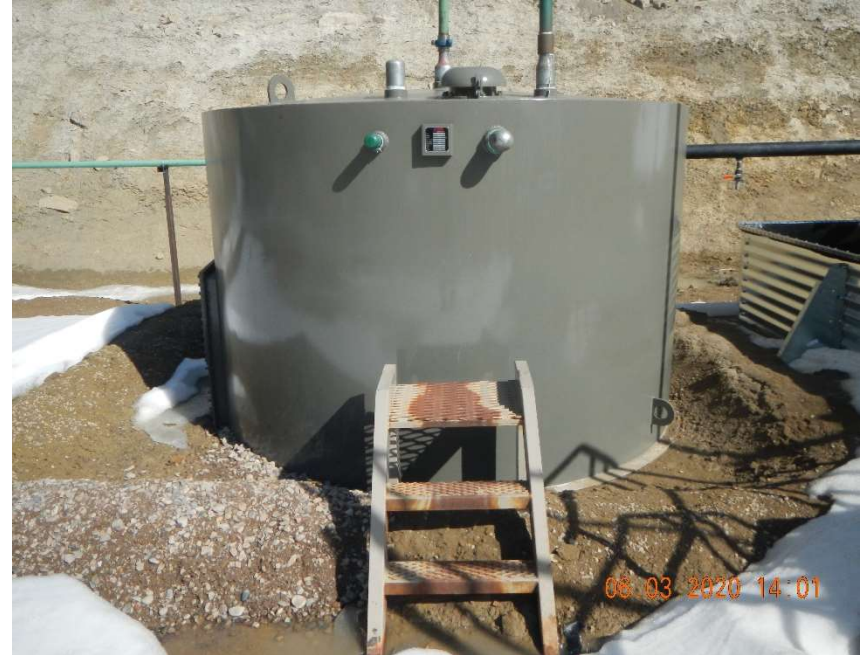
Unlabeled steel AST, secondary containment in disrepair.
