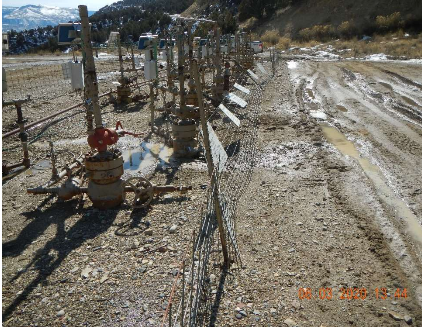
Wildlife fencing around wellheads in disrepair, vehicle tracking on location and fluids pooling around wellheads.
