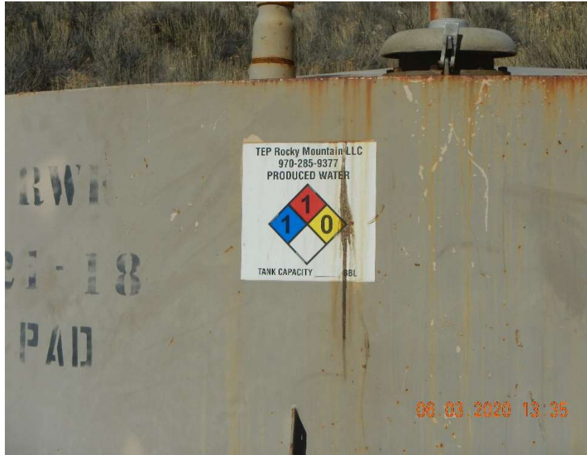
Produced Water steel AST missing capacity label.
