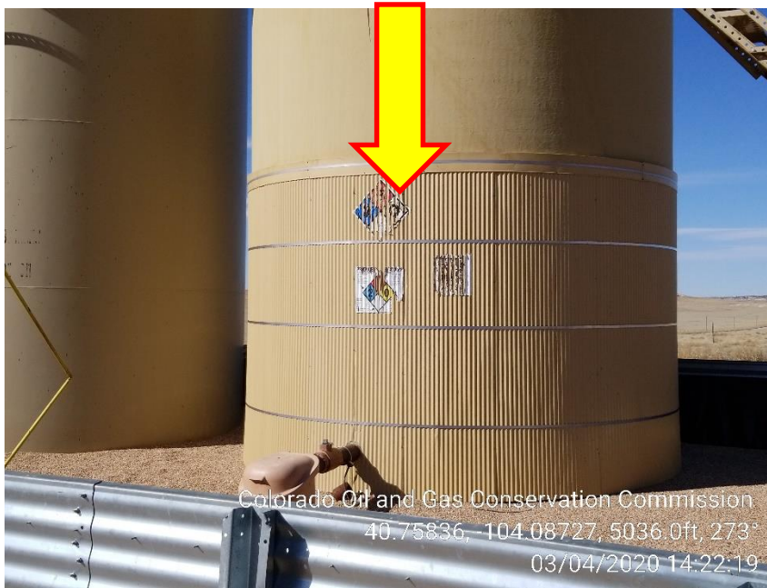
Photo 3 – Produced Water Tank – Missing Content and Capacity and NFPA Label has faded.
