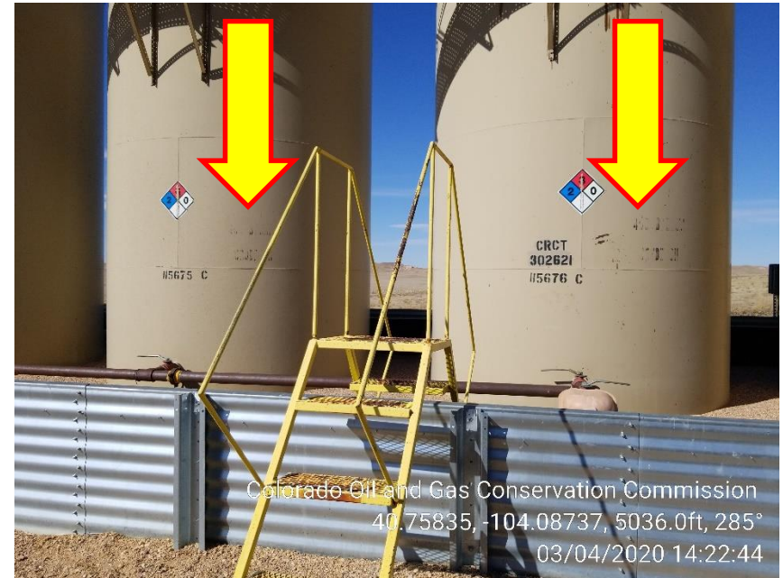
Photo 4 – 2 Middle Tanks – Missing Content and Capacity
