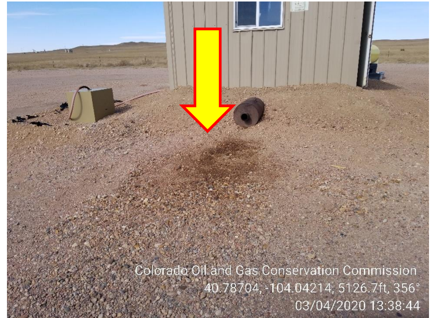
Photo 4 – Stained Soil at Exhaust
