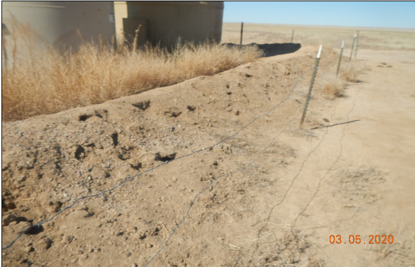
Photo 3. The berms at the tank battery has holes and is degraded. The fence around the tank battery is not maintained.
