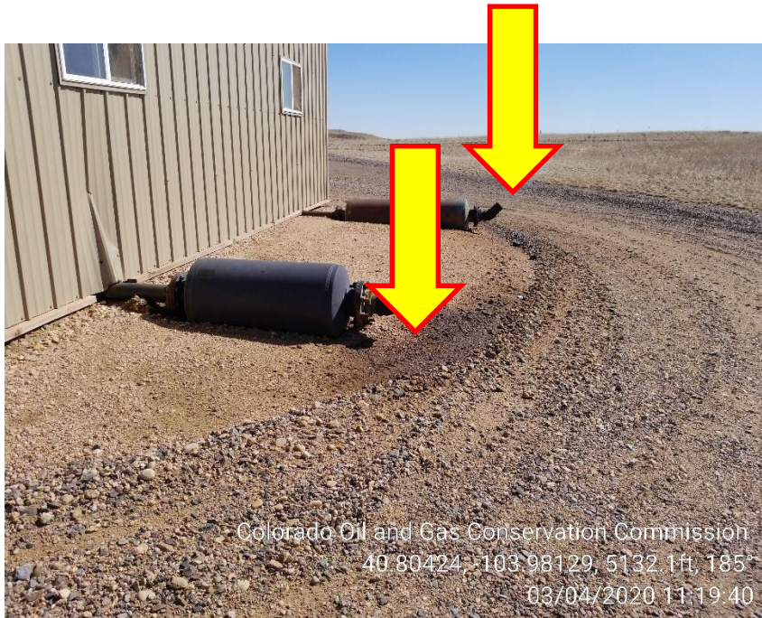
Photo 3 – Stained Soil at Engine Exhaust
