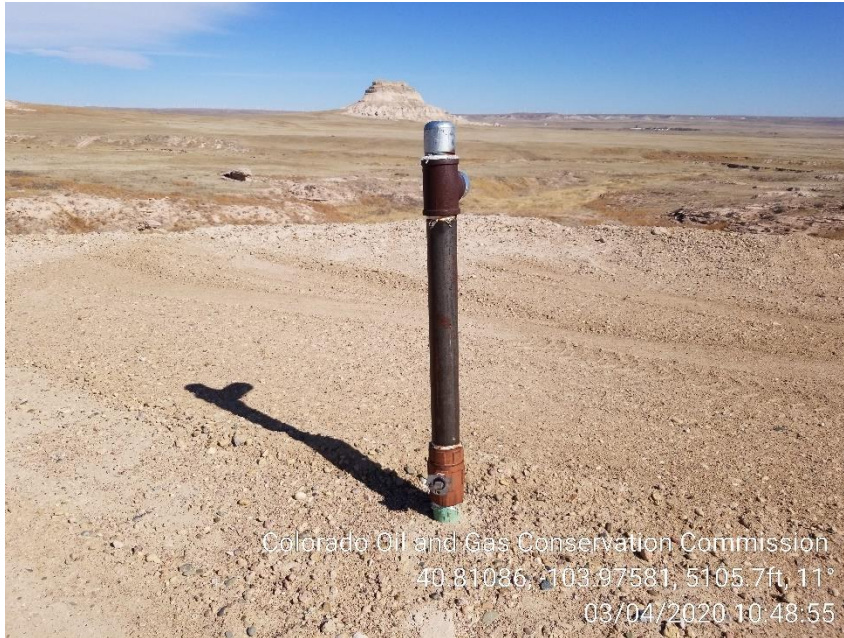
Photo 3 – Unmarked Riser in the NE Corner of Location
