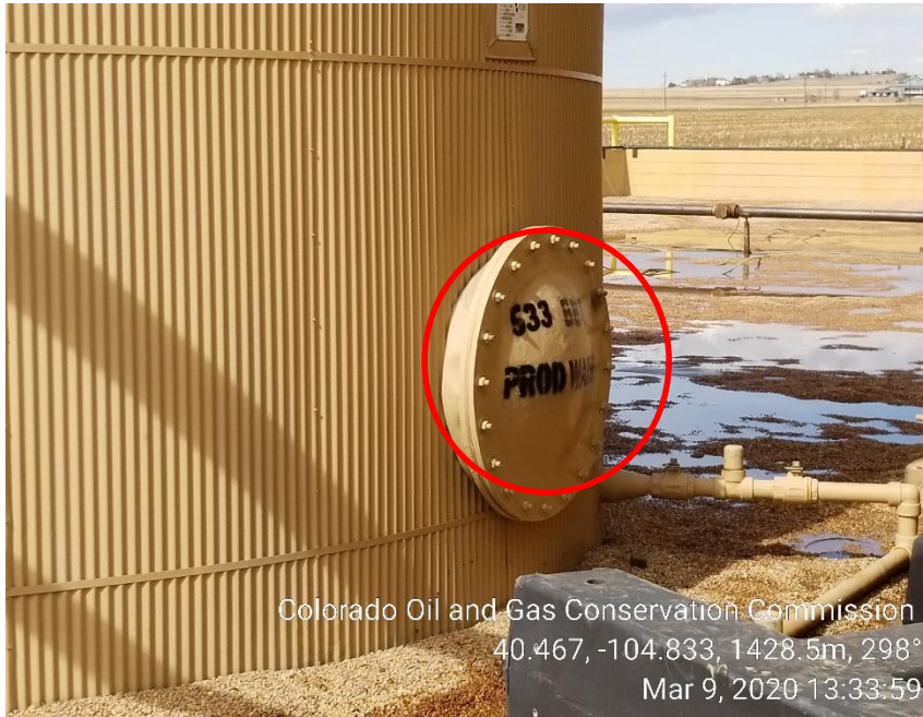
Photo 27: No NFPA placard/labeling on wrong side of tank.
