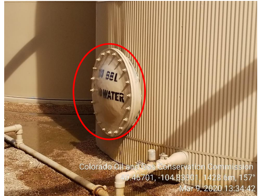
Photo 28: No NFPA placard/labeling on wrong side of tank.
