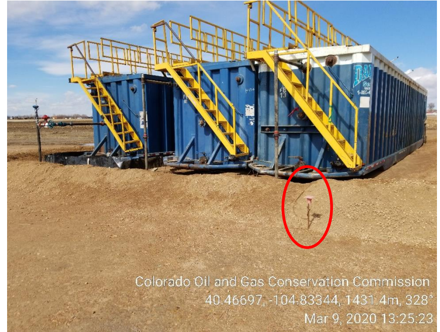
Photo 20: Tanks appear to be grounded
