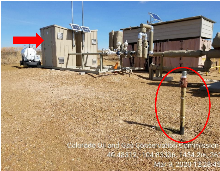
Photo 31: Disconnected gas meter house/unused riser
