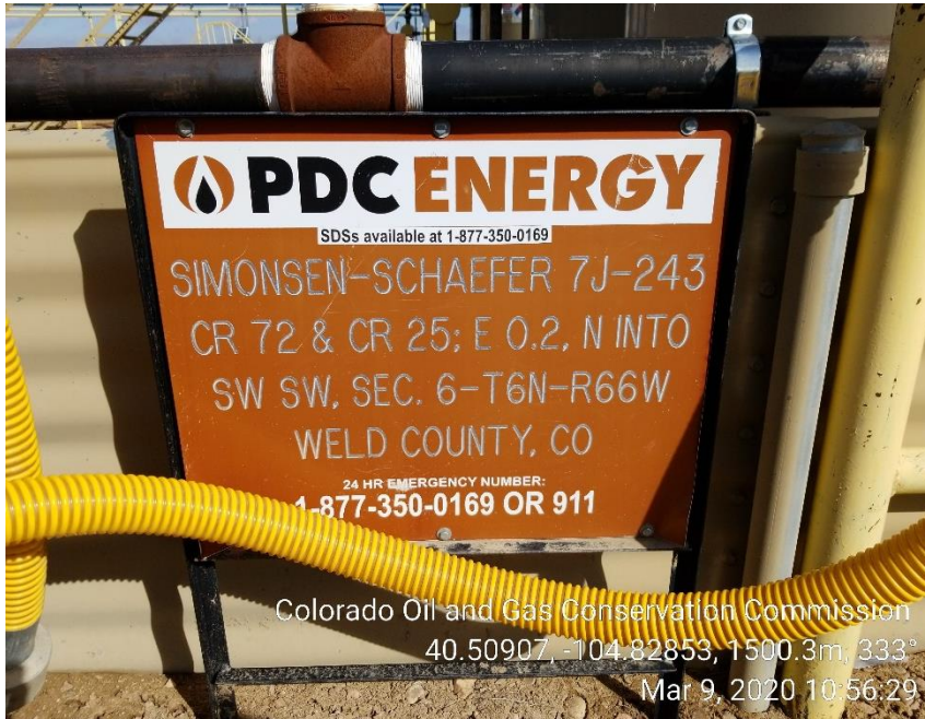
Photo 1: Tank Battery Sign
