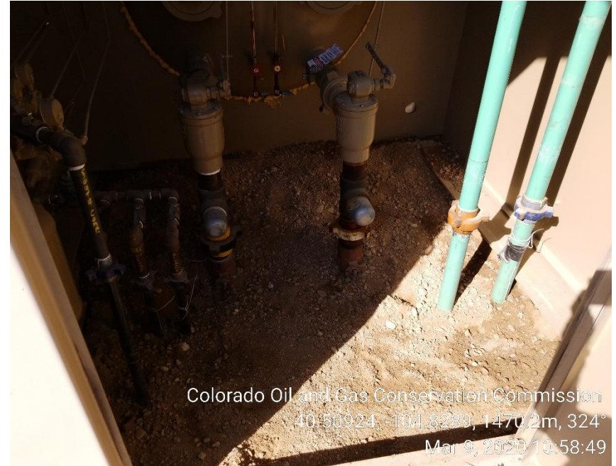
Photo 4: Stained soil removed
