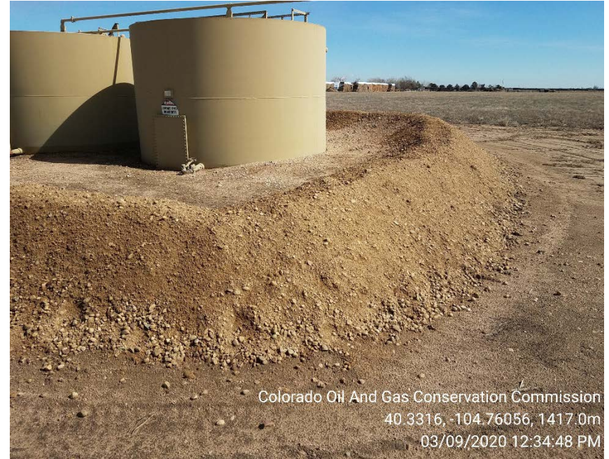
Crude oil tank berm on 3/9/2020
