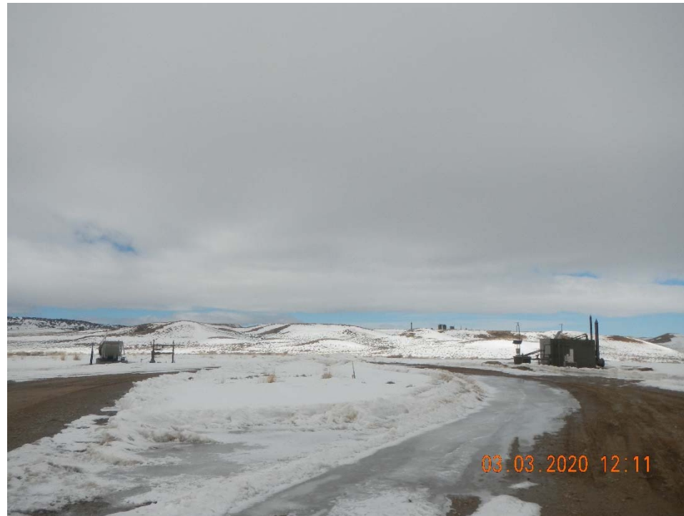
Photo 1. Overview of location taken facing southwest.
