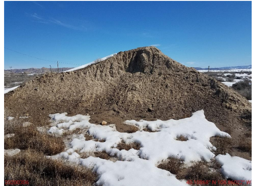
Photo 4: Photo taken from the south end of the Location, facing east. Photo shows soil stockpile is not protected in accordance with 1002.c; erosion degradation evident.
