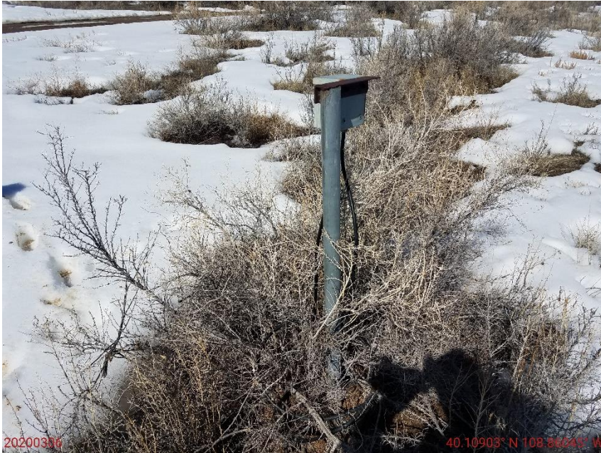
Photo 5: Photo taken from the north end of the Location. Photo shows what appears to be an electrical box; cables have been disconnected (see photo 6); Equipment is unused and needs to be removed in accordance with 603.f.
