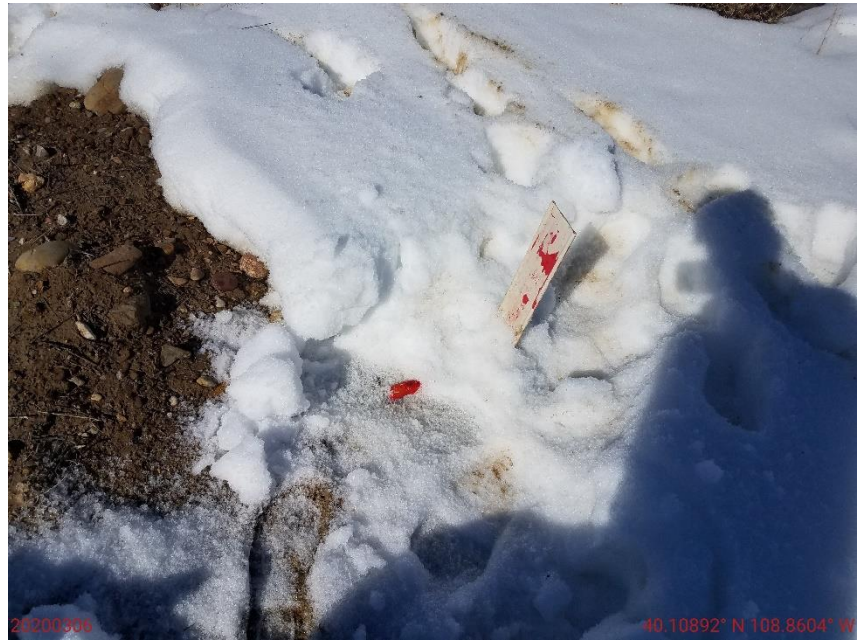
Photo 2: Photo taken from anchor on the northeast corner of the Location. Rule 1003.a requires anchors to be identified by a marker of bright color not less than 4 feet in height. Markers in disrepair.
