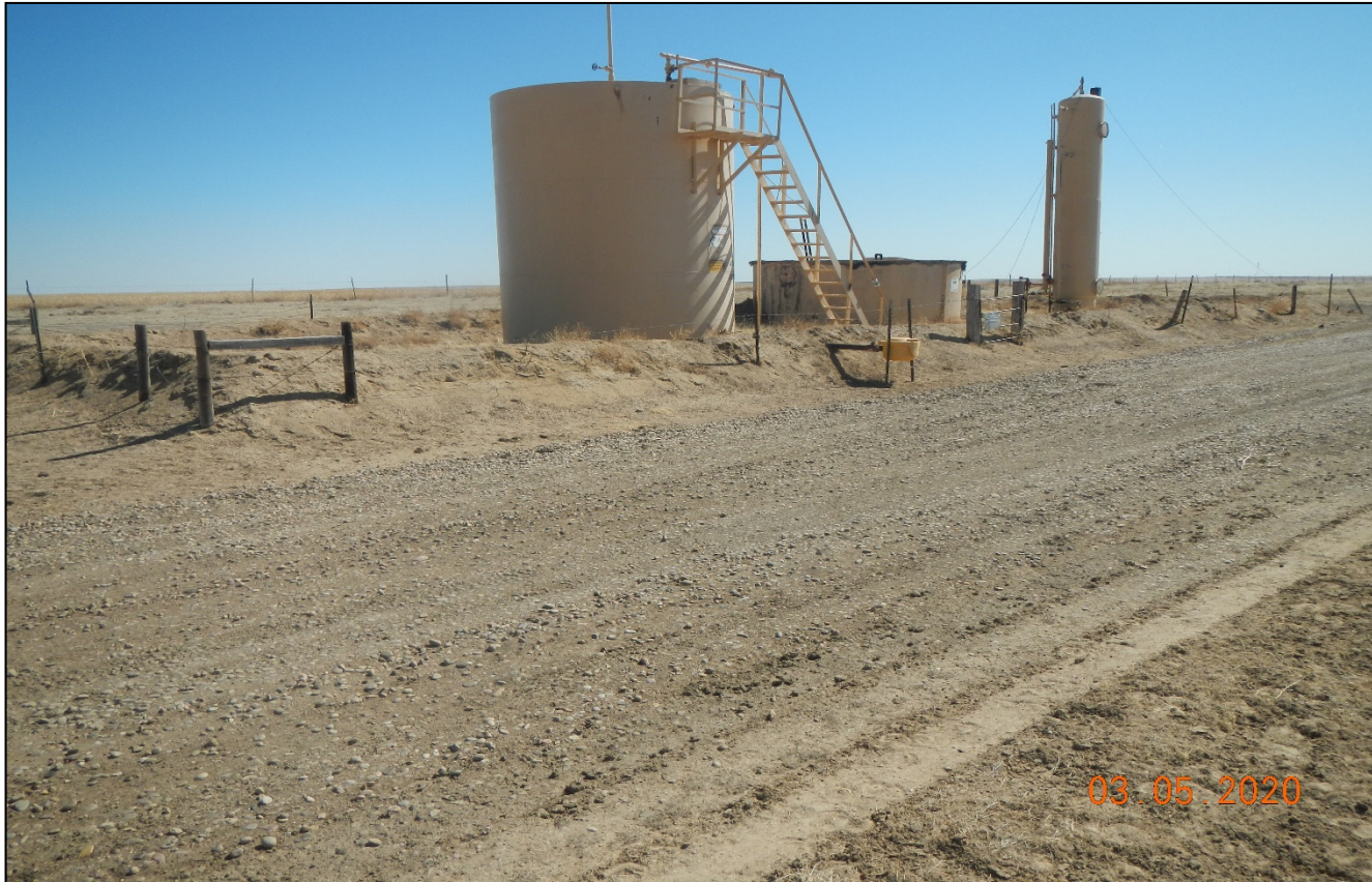
Photo 2. Facing toward the tank battery. The fence around the battery is maintained and secondary containment has been installed at pipe outlet.
