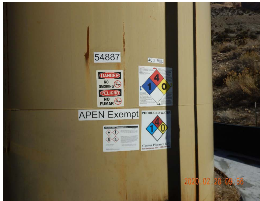
Photo #3 – Tank battery labels and placards.
