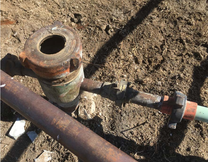
Wellhead. No evidence of gas leakage. Meter gas readings non-detect.
