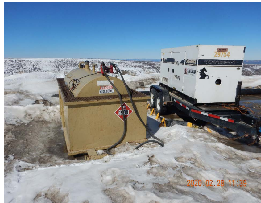
Photo #44 – 1000 gallon dyed diesel AST inside of secondary containment device located in northwest corner of pad along with generator.
