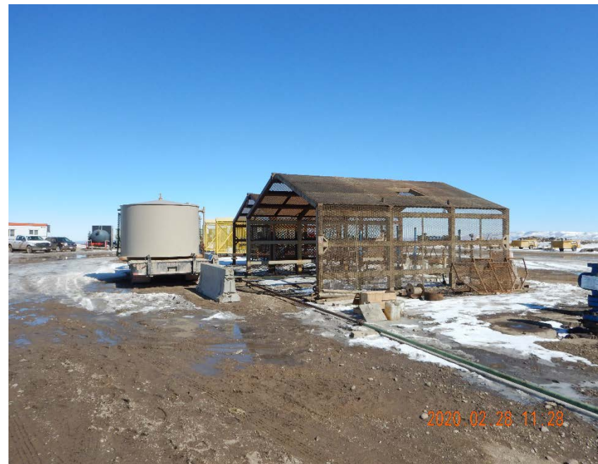
Photo #34 – AST on trailer located west of wellheads was plumbed to surface lines on inspection date. AST did not have any secondary containment devices installed.
