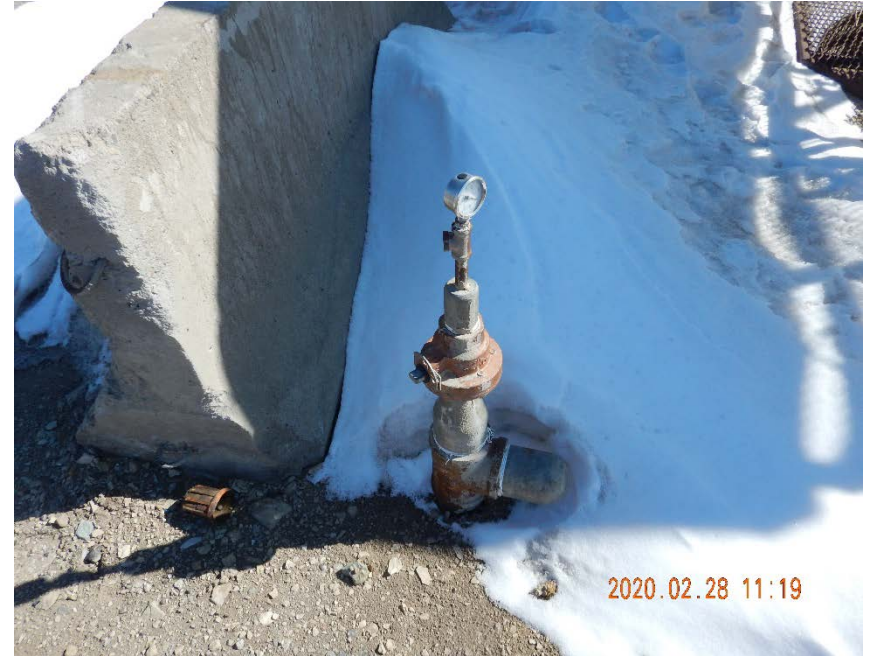
Photo #12 – Unmarked flowline riser located NW of wellheads.
