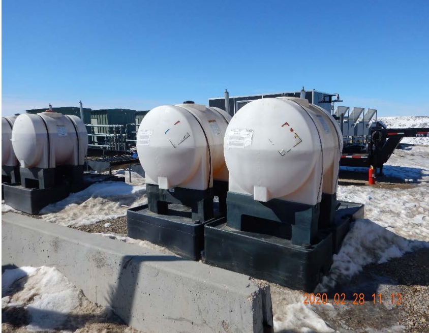
Photo #3 – NFPA placards on day tanks were damaged and tank labels were faded on inspection date.
