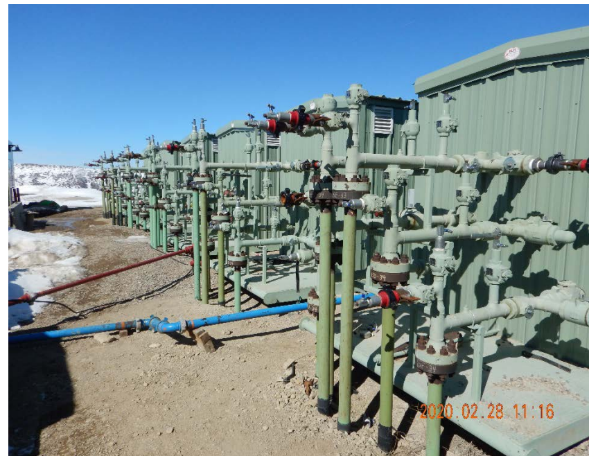
Photo #10 – Flowline risers at meter sheds located on north side of pad.
