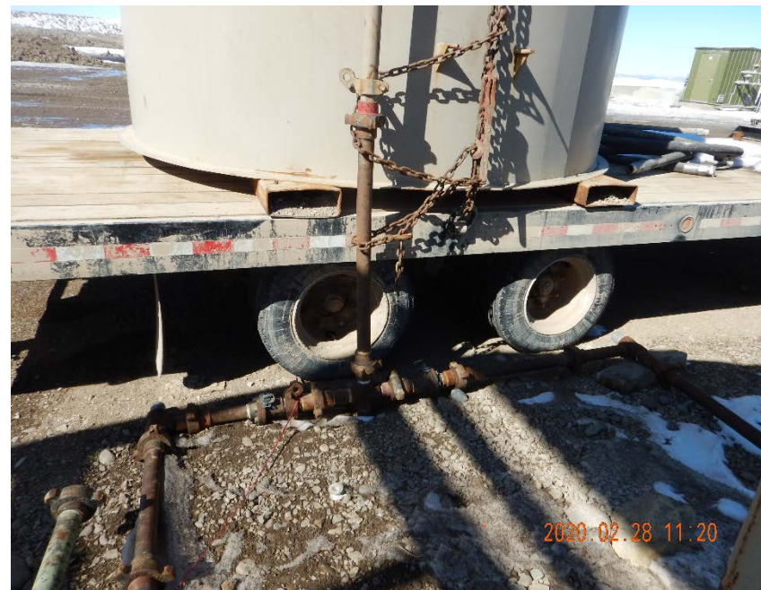
Photo #36 – Close-up of surface flowlines lined to 80 bbl produced water AST lacking secondary containment device.
