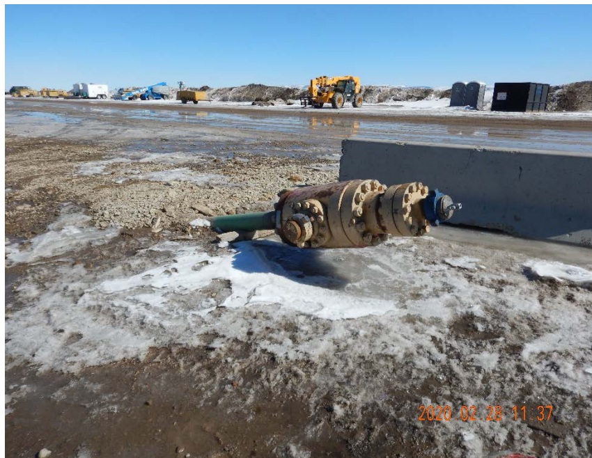
Photo #43 – Unmarked, angled flowline daylights southeast of wellheads.
