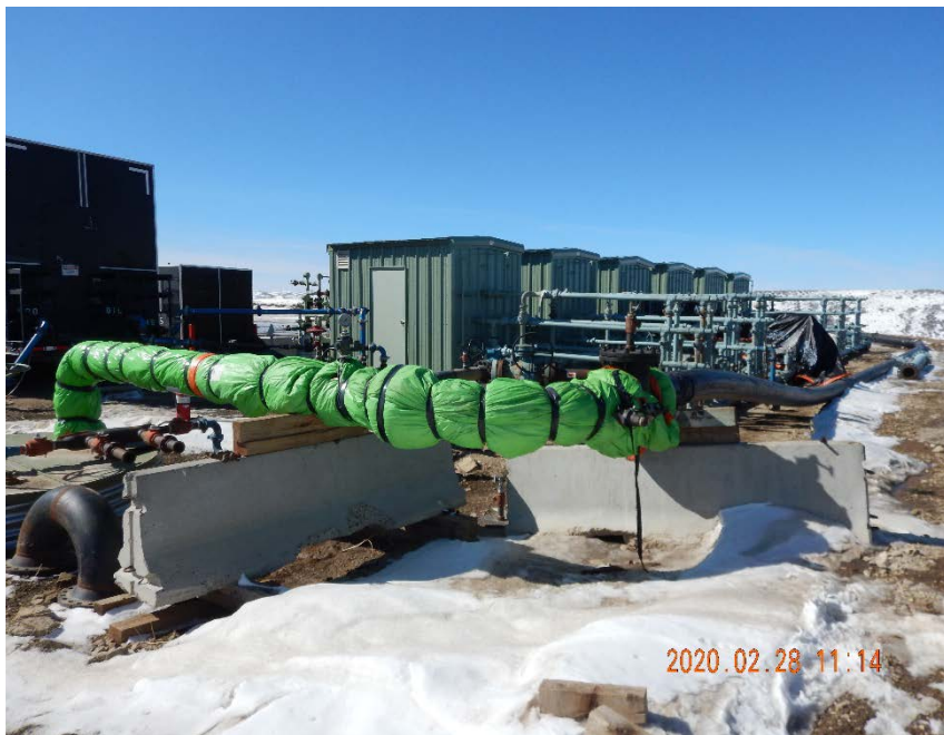
Photo #5 – HDPE surface line and gas meter sheds with flowline risers located on north side of pad.
