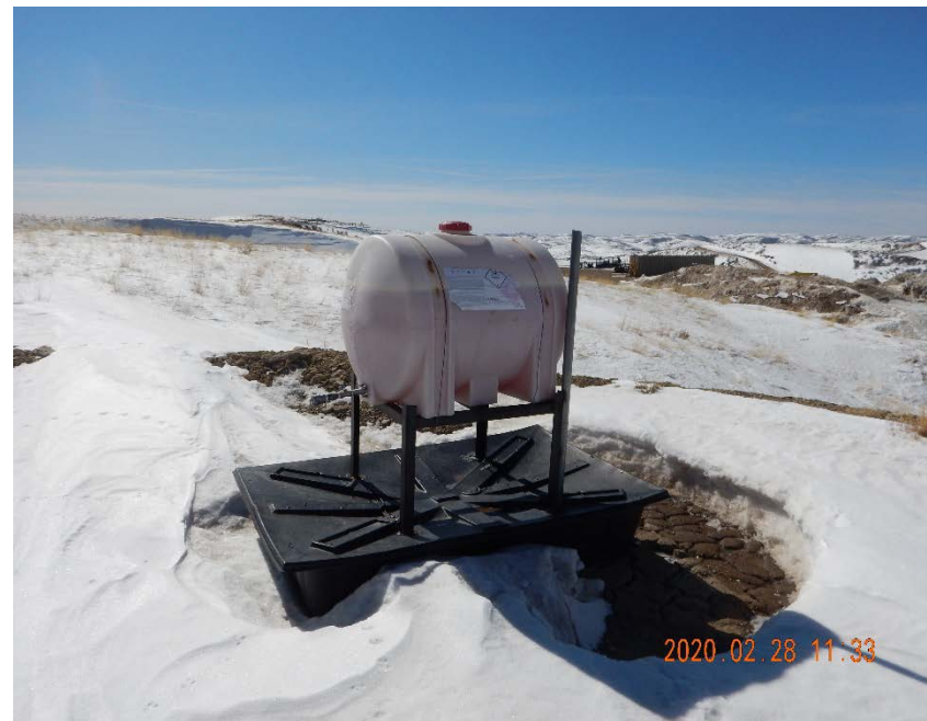
Photo #42 – Chemical storage day tank with secondary containment device located in southwest corner of pad. Note that tank label is faded and damaged.
