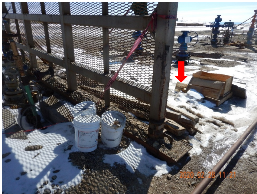
Photo #13 – Chemical storage buckets and wood debris located on west side of wellhead area. Note overturned chemical storage container marked by red arrow.
