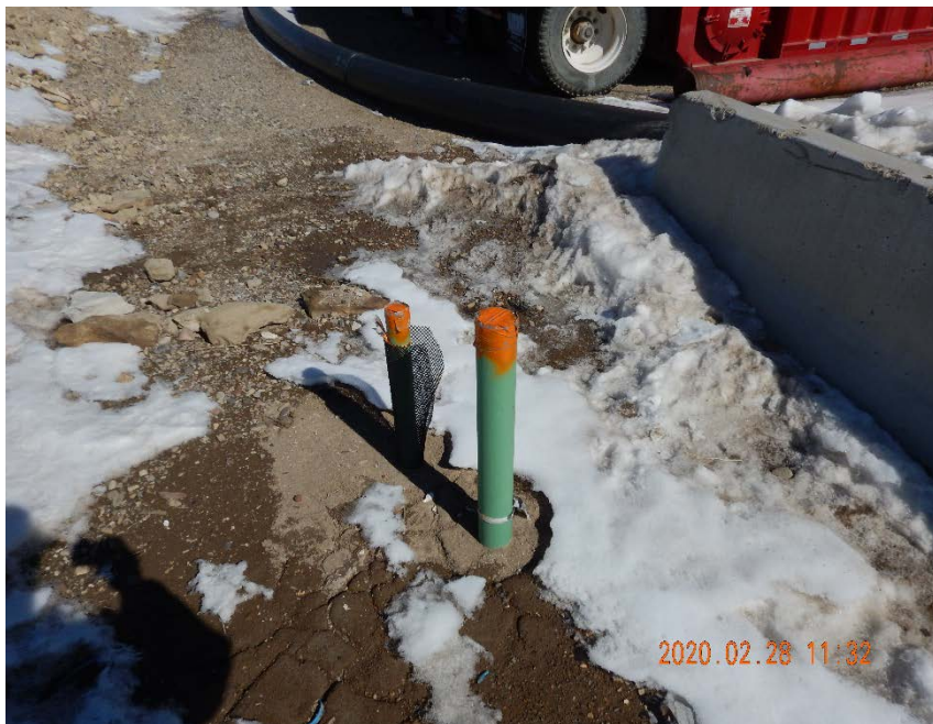
Photo #41 – Marked, uncapped flowline risers located southwest of frac tanks.
