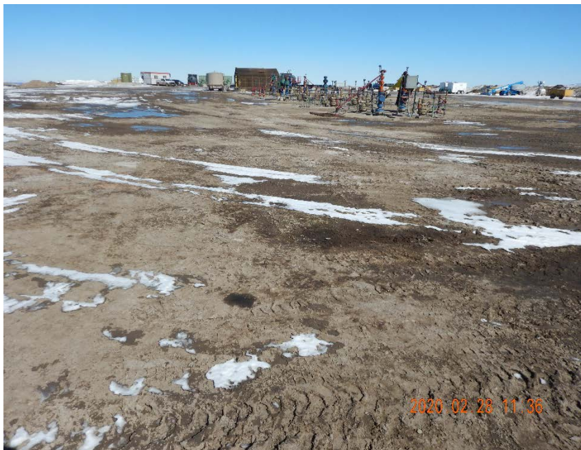
Photo #29 – Localized accumulations of oil-stained soil on south side of pad.
