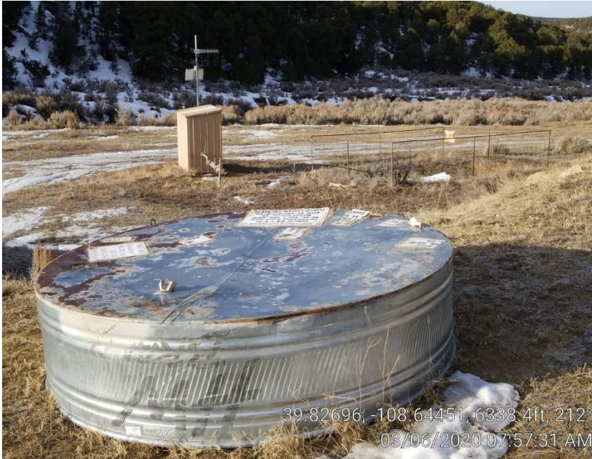
Photo 2. Unused tank near gas meter pit
