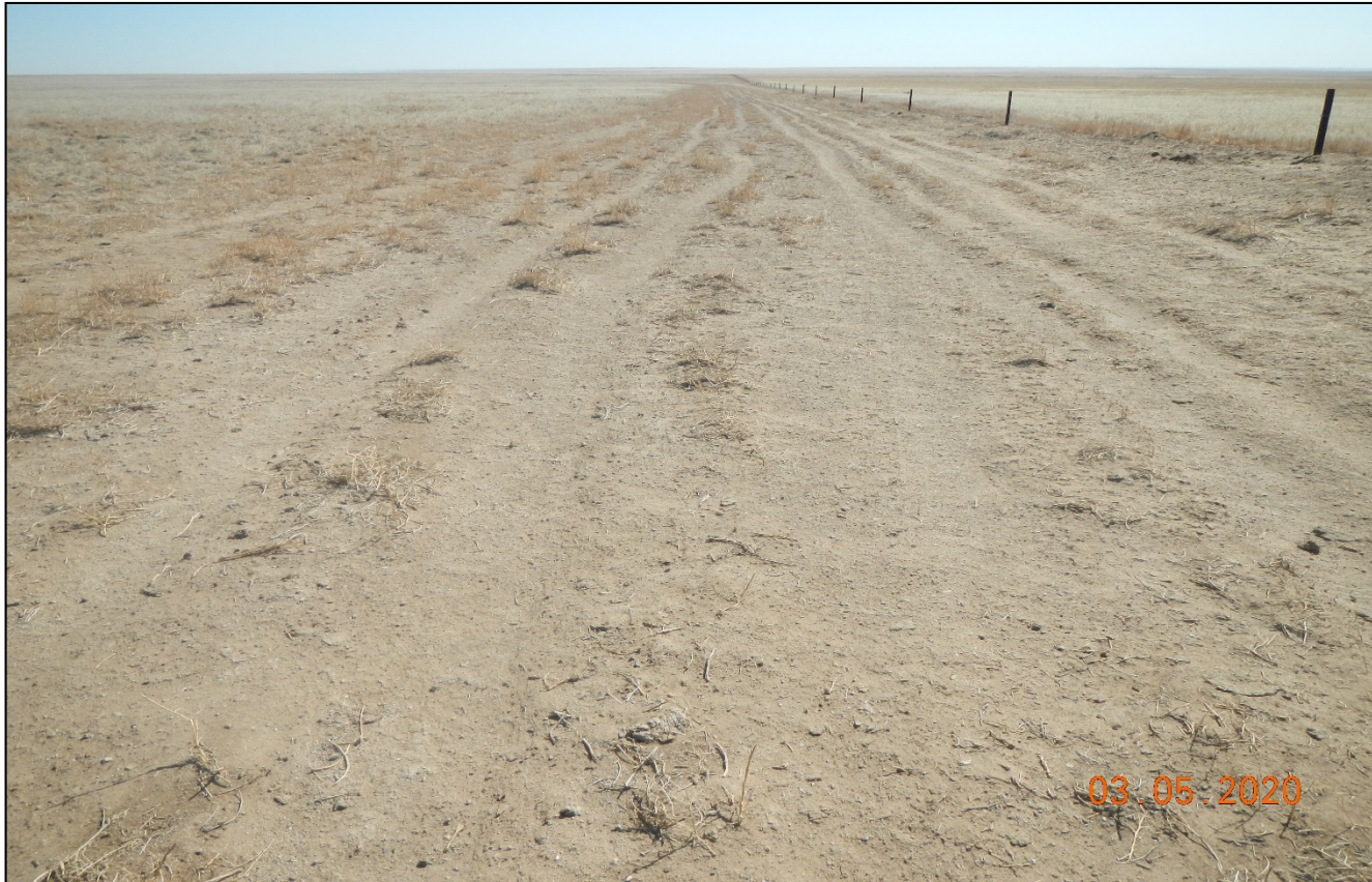
Photo 3. Facing south along the former access road. The access road is bare of vegetation and there is signs of wind erosion occurring.
