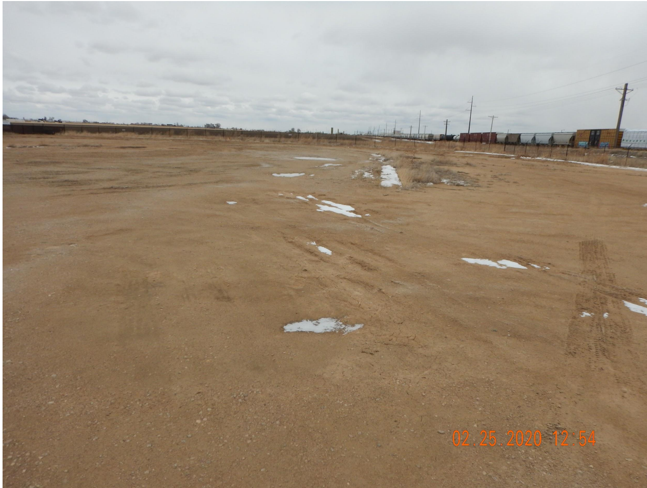
Photo 1. Photo taken from the well and tank battery location, facing East. Photo illustrates Operator has removed all the major equipment but has not conducted surface reclamation (i.e., remove gravel, contour, ect...).
