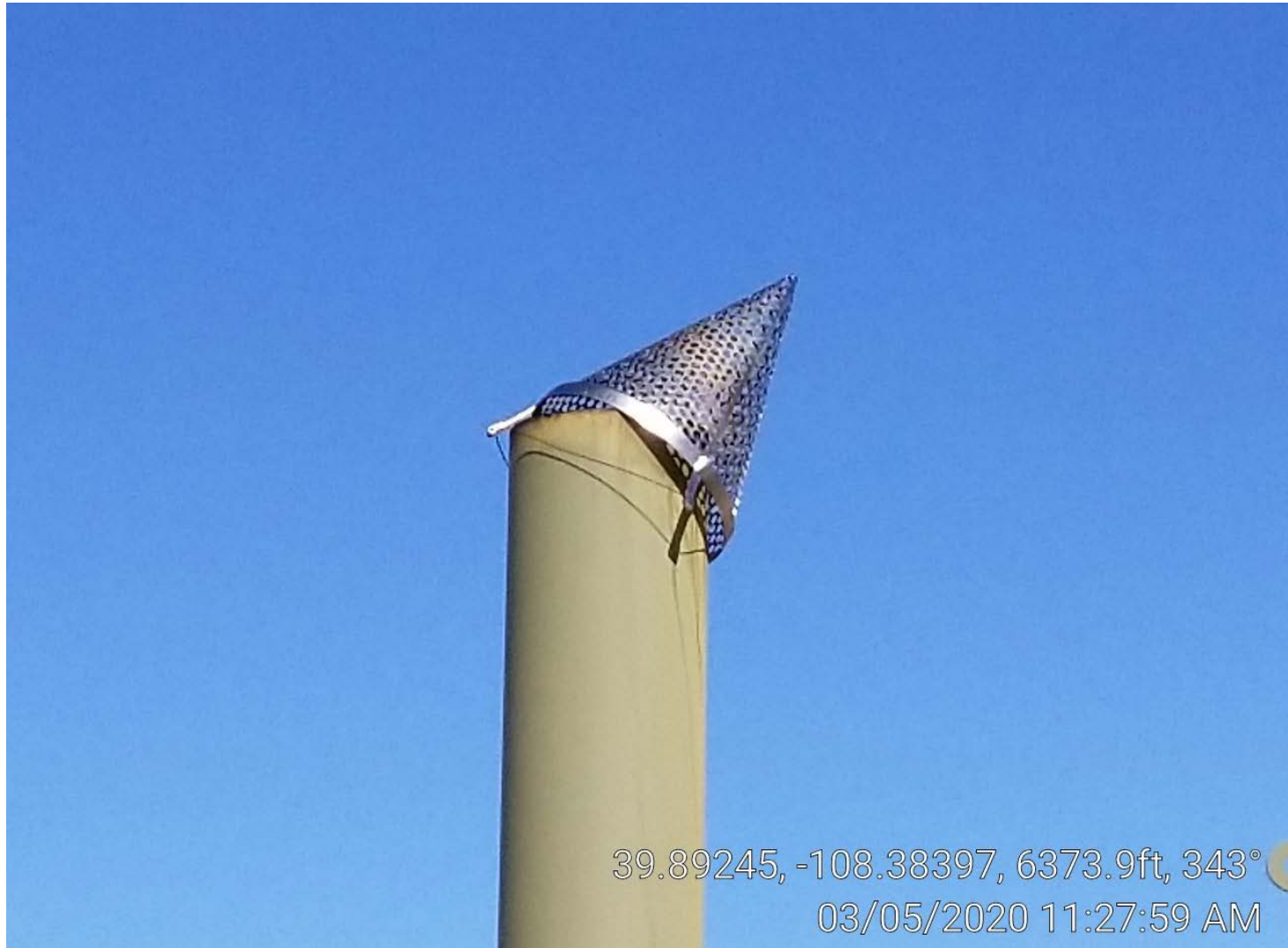
Photo 5. Separator bird cone.
