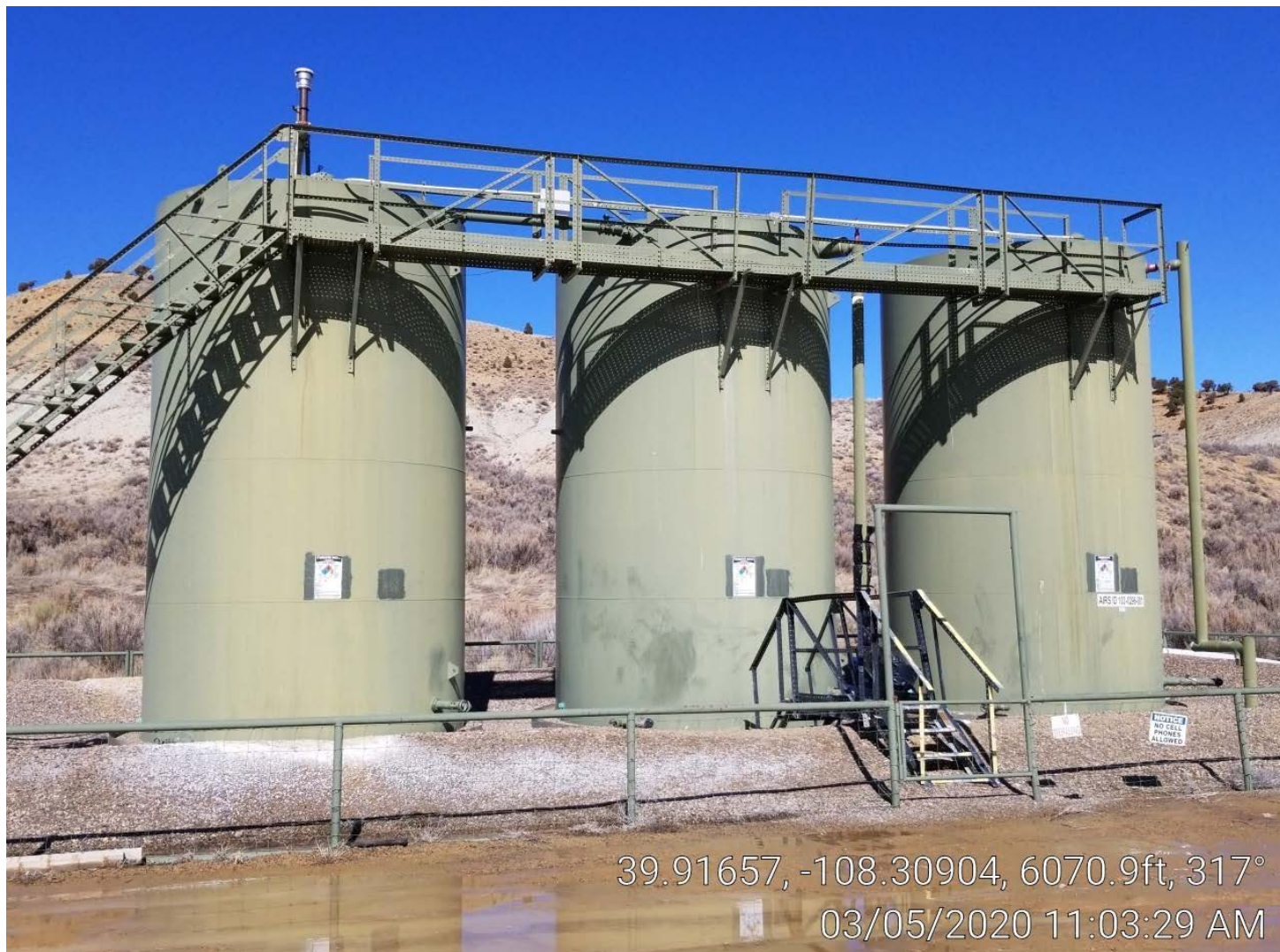
Photo 3. Tank battery.
