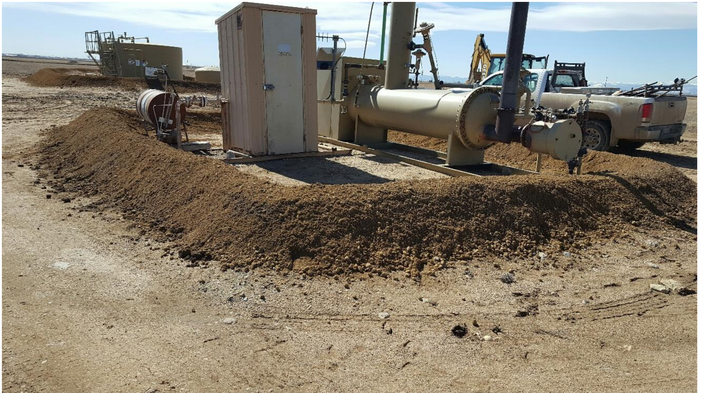
Figure #1 Berms have been repaired.
