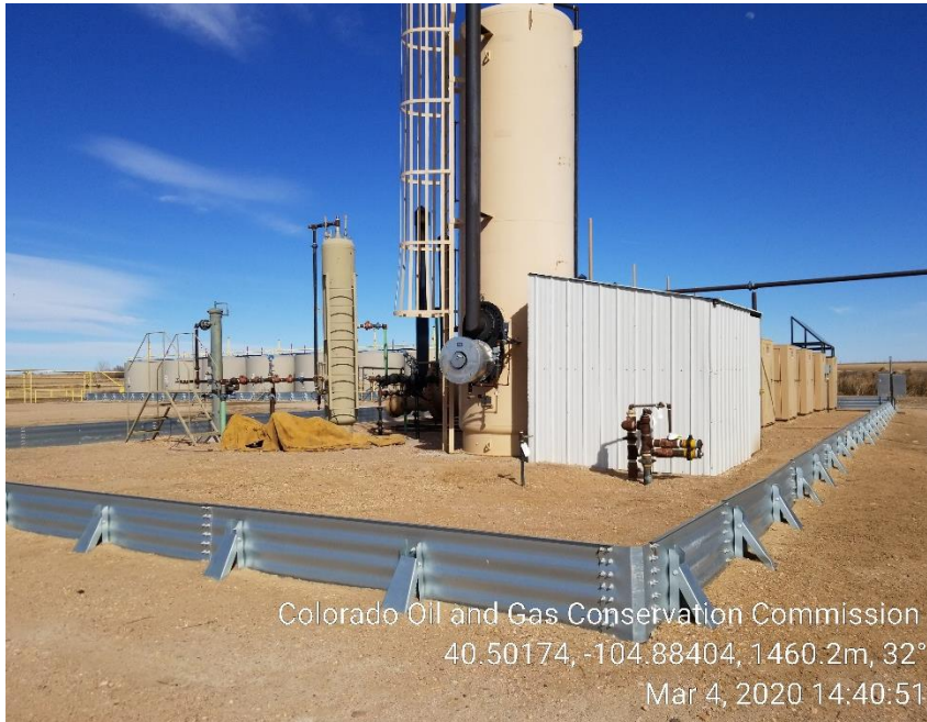
Photo 13: Heater treater removed, risers LO/TO
