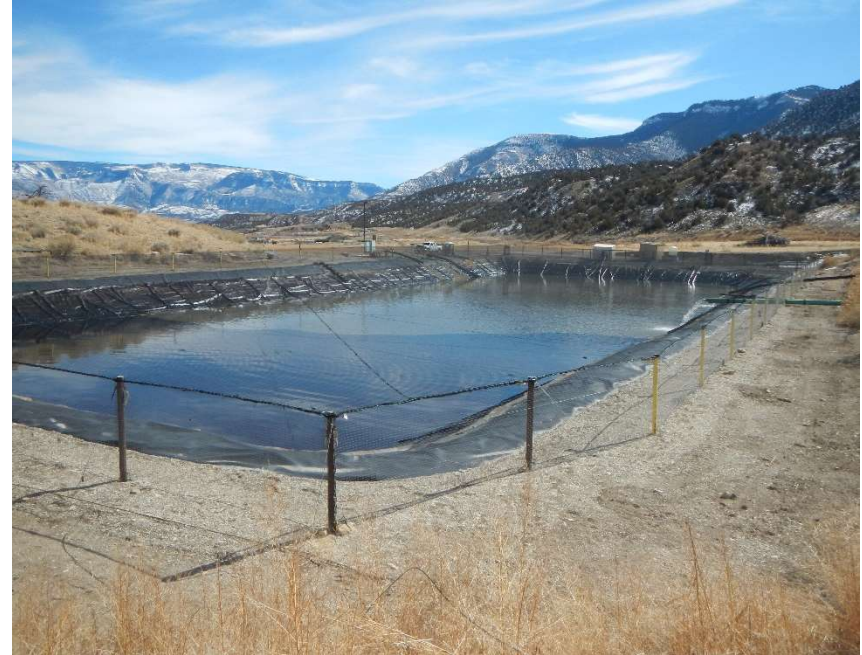
Free product present on ~20% of the pit fluid and liner.
