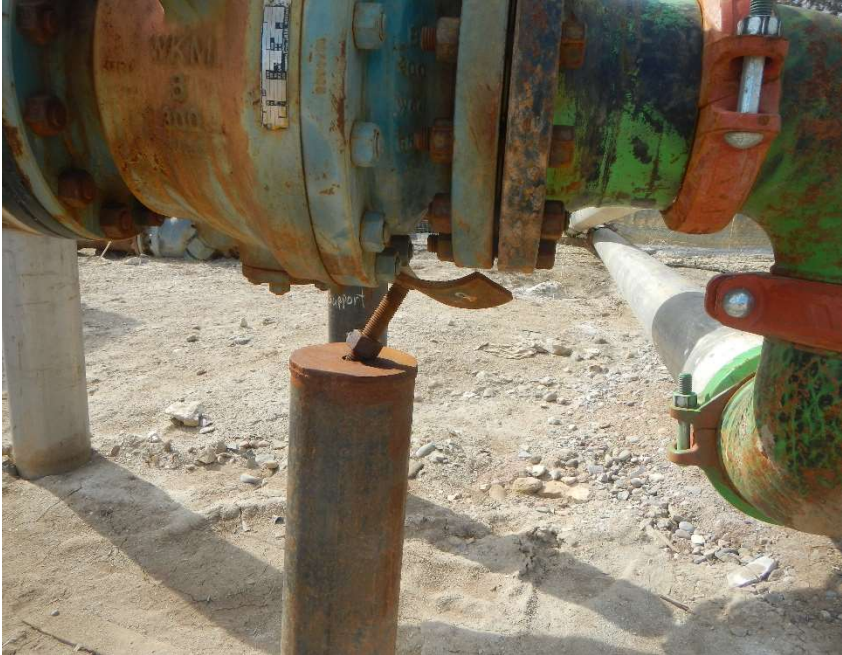
Flow line support in disrepair.
