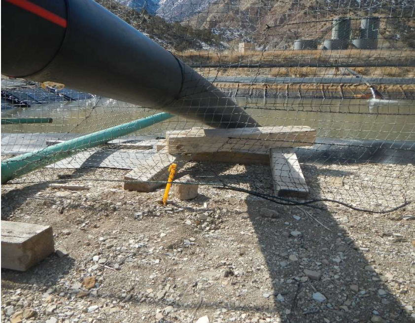
Gaps in the base of the wildlife mesh on the east side of the pit. Note that pipe support cribbing is in disrepair.
