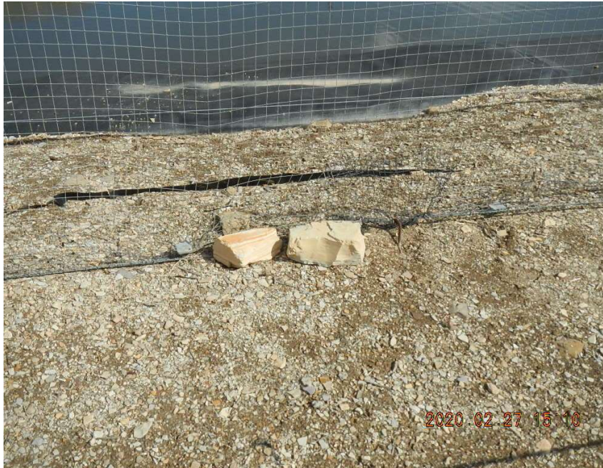
Gaps in net secured with rocks.
