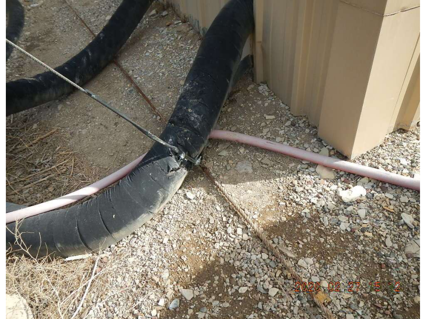
Net support guy wire wearing through pipe insulation and pipe.
