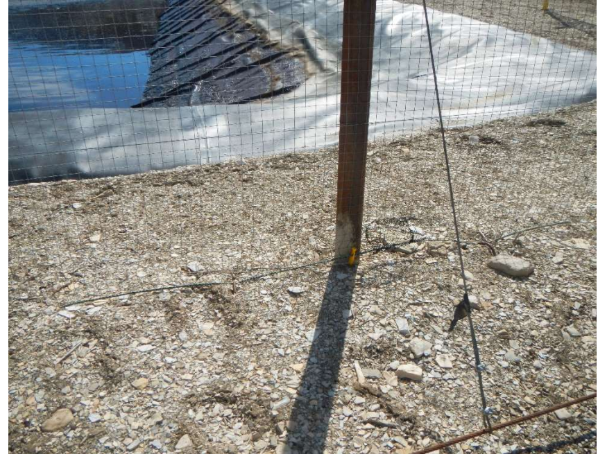
Gaps in the base of the wildlife mesh on the east side of the pit.
