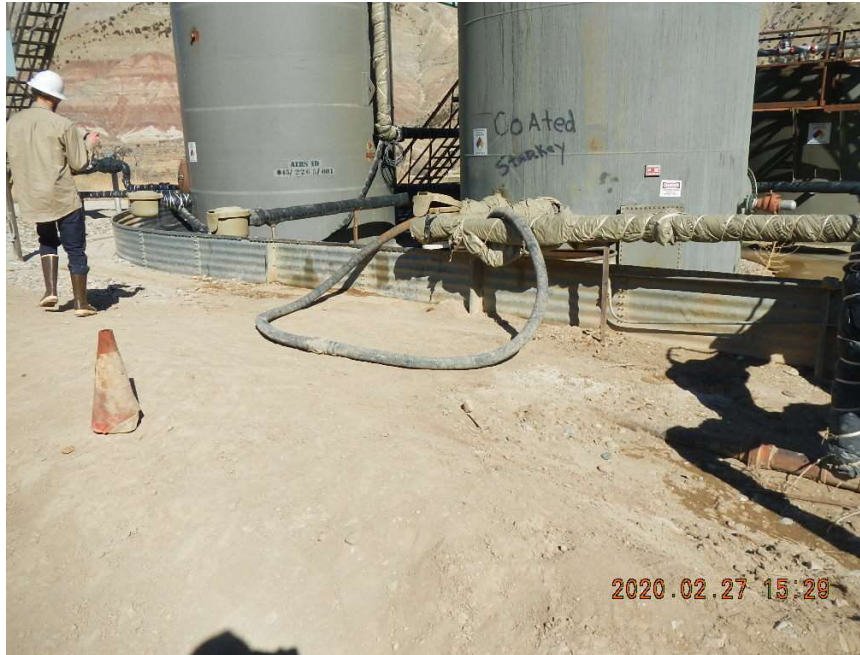
Load out hose draped over equipment, staining on the exterior of the tank battery secondary containment.
