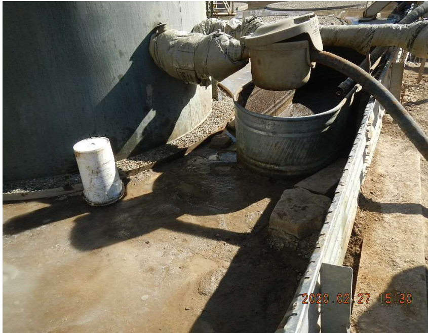
Potential impacted fluids within the tank battery secondary containment.
