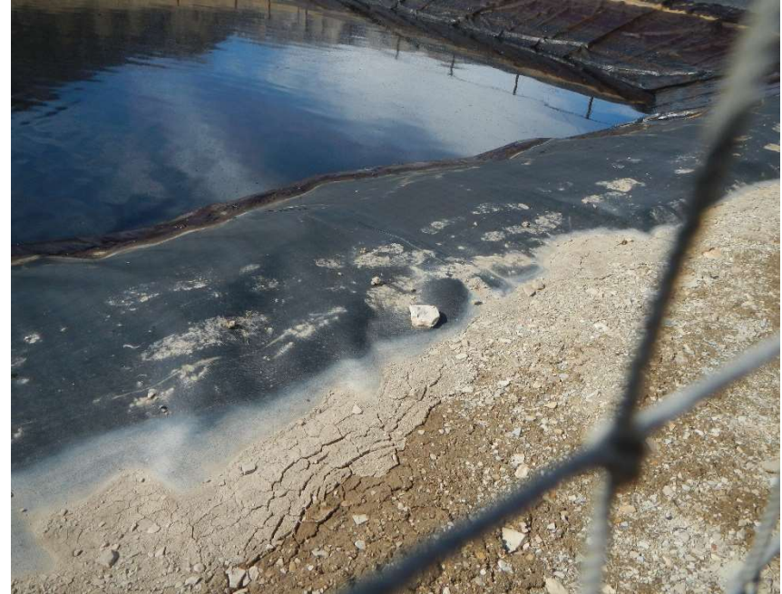
Sediment encroaching on pit liner.
