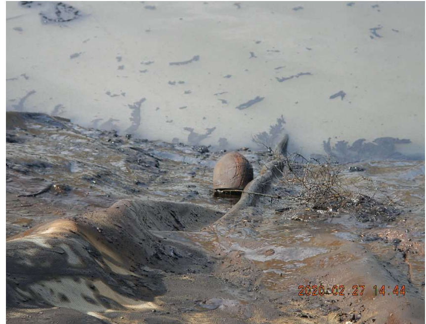
Trash and debris on pit liner within the pit.
