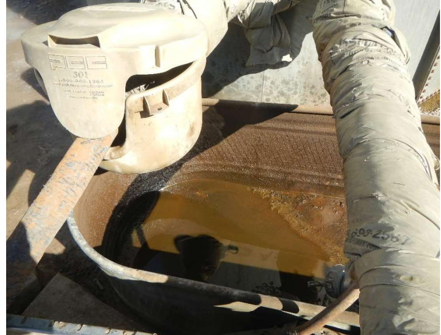
Photo #18 – Trough containing potential impacted fluid located beneath the tank battery load out.
