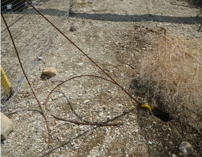
Subsidence around rig anchor supports on the west side of the pit.
