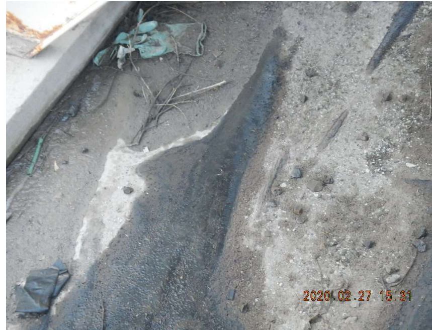
Trash and debris within the tank battery secondary containment.
