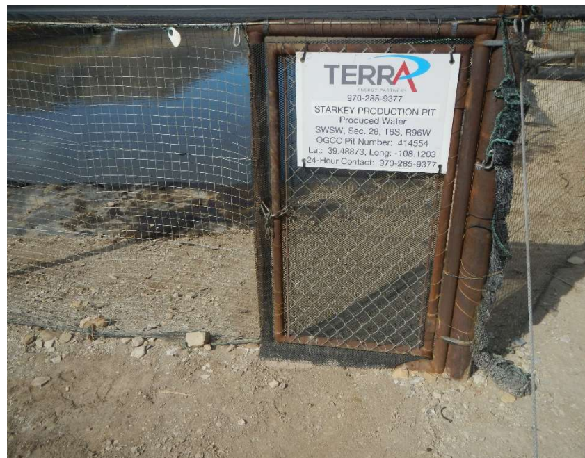
Starkey Production Pit sign. Note oil accumulation on upper pit liner and soil at the southeast corner of the pit.
