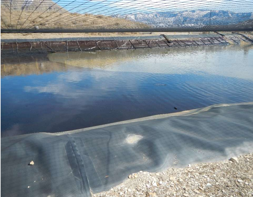
Free product present on of the pit fluid (~20%) and liner.
