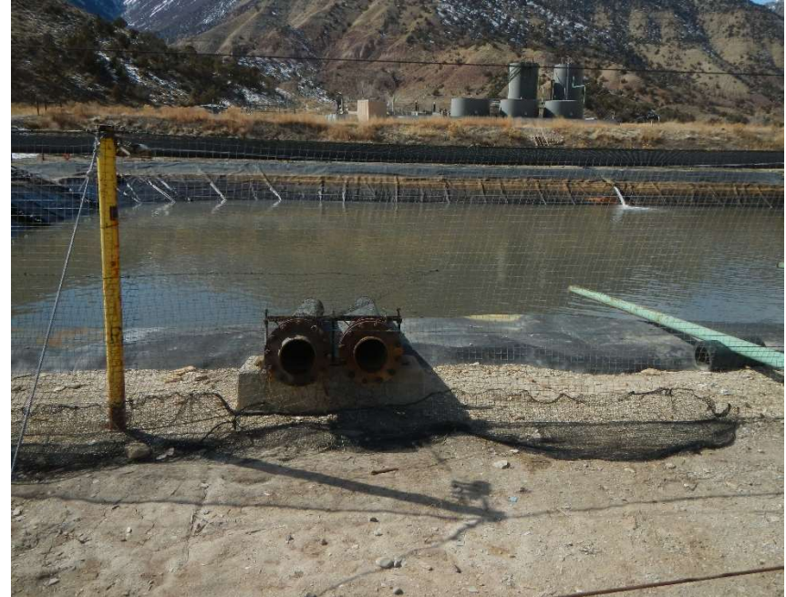
Uncapped manifold on the eastern side of the pit.
