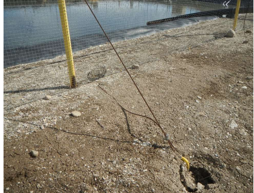
Subsidence around rig anchor supports on the west side of the pit and the netting support bollards leaning towards the east.
