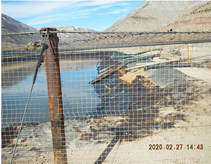
Hoses and poly line resting directly on the pit liner.
