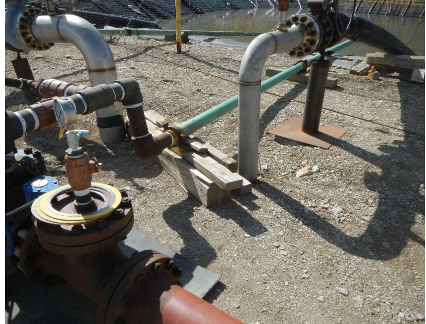
Flow line cribbing and support in disrepair.
