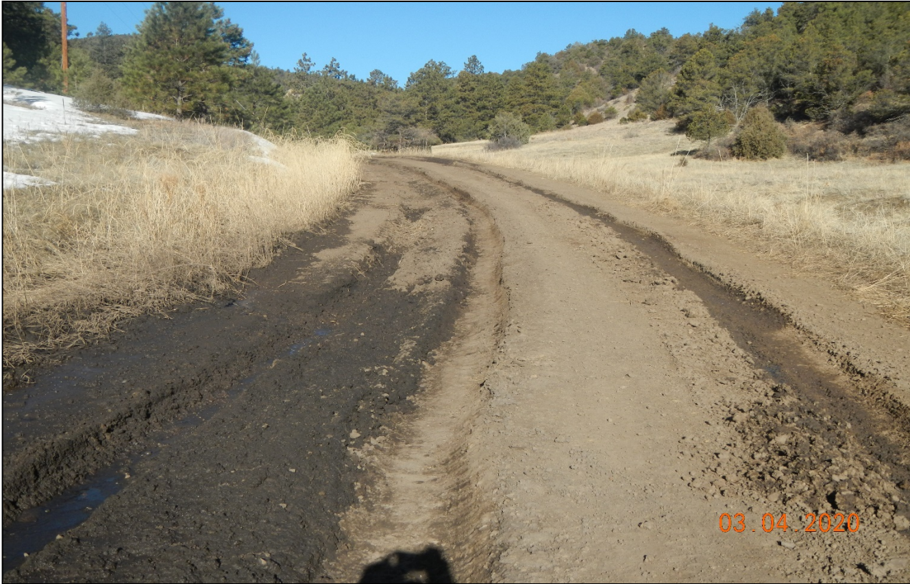
Photo 1. Facing northwest along the main lease road toward the location. The road has deep ruts and is not being maintained.
