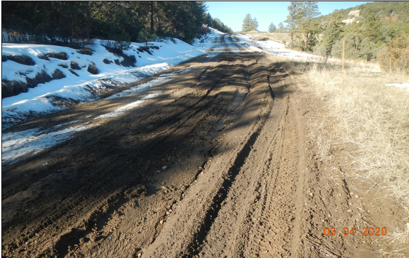
Photo 2. Facing northwest along the main lease road toward the location. The road has deep ruts and is not being maintained.
