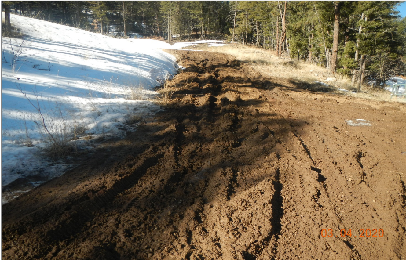
Photo 2. Facing southwest toward the access road. The road has deep ruts and is not being maintained.
