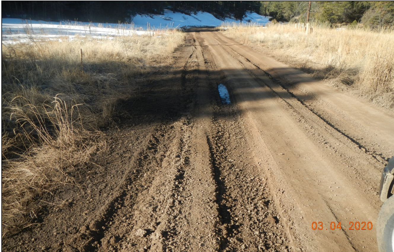
Photo 1. Facing west along the main lease road in Alamosito Canyon. The road has vehicle rutts and is not being maintained.
