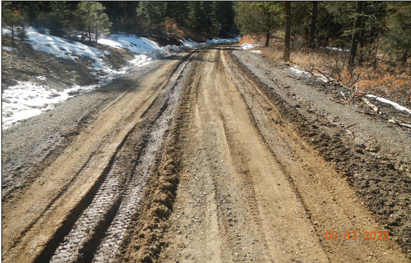
Photo 3. Facing southwest as it ascends the hillside The road has deep ruts and is not being maintained.
