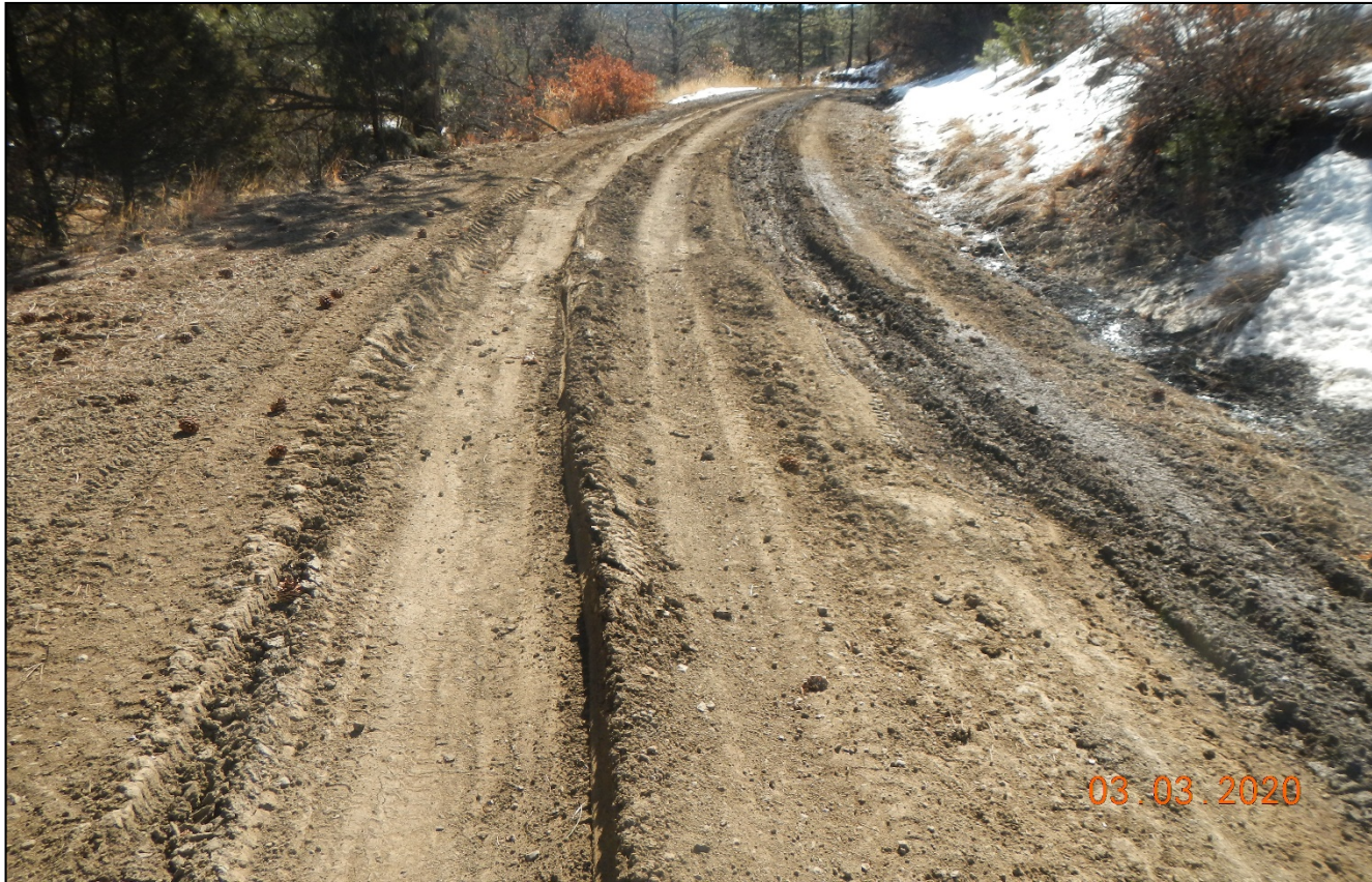
Photo 1. Facing southeast through Little Bingham Canyon. The road has deep ruts and is not being maintained.
