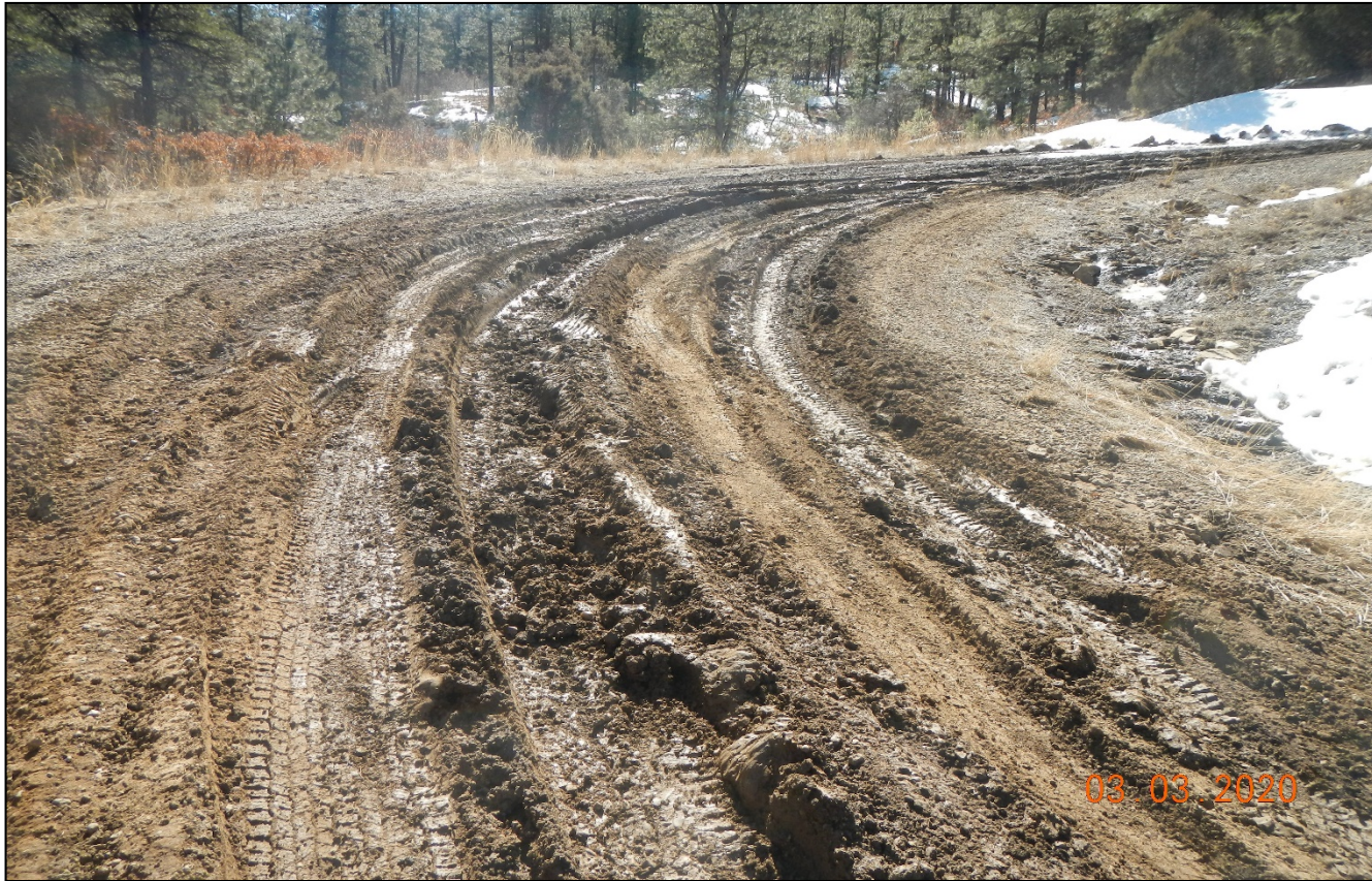
Photo 2. Facing south through Little Bingham Canyon. The road has deep ruts and is not being maintained.
