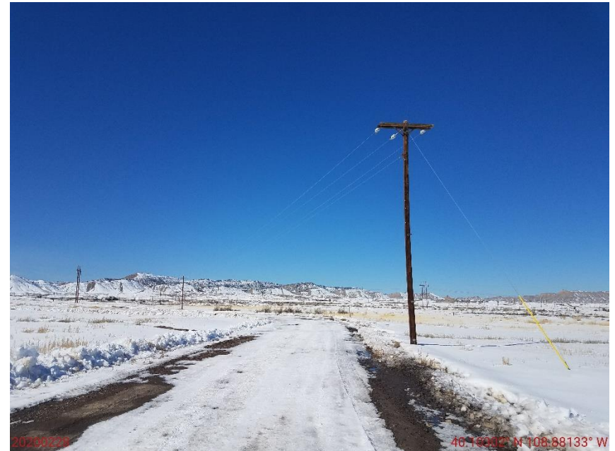
Photo 4: Photo taken from the west end of the Location, facing west. Photo shows the Oil and Gas utility pole on Location, and poles leading to the Location, have not been removed pursuant to Rule 1004.a
