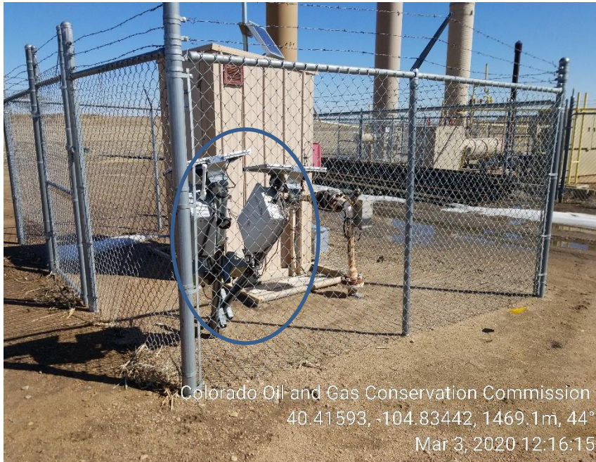
Photo 3: Unused equipment; disconnected gas meter house
