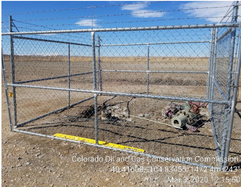
Photo 1: Wellhead; unused equipment, no sign
