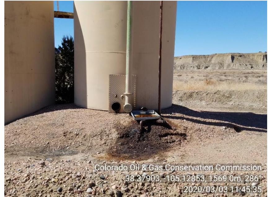
PHOTO 6: A BULLPLUG ON 210 BBL TANK IS LEAKING. THERE IS AN AREA OF IMPACTED SOIL APP. 3' BY 6' NEAR LEAKING PLUG. CALLED CONTACT NUMBER POSTED ON BATTERY SIGN AND HAD TO LEAVE A MESSAGE. Securely fasten all valves, pipes, and fittings to ensure good mechanical condition, inspect at regular intervals and maintain in good mechanical condition per Rule 605.d. Properly treat or dispose of oily waste in accordance with 907.e."
