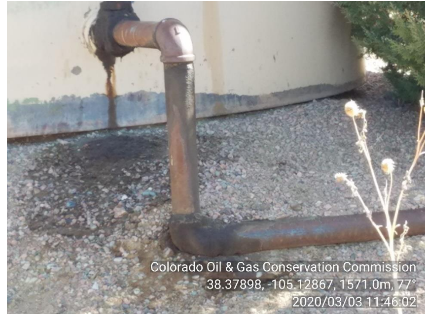
PHOTO 8: VALVE ON 210 BBL TANK IS SEEPING. THERE IS AN AREA OF IMPACTED SOIL APP. 3' BY 1' NEAR SEEPING VALVE.. Securely fasten all valves, pipes, and fittings to ensure good mechanical condition, inspect at regular intervals and maintain in good mechanical condition per Rule 605.d. Properly treat or dispose of oily waste in accordance with 907.e.
