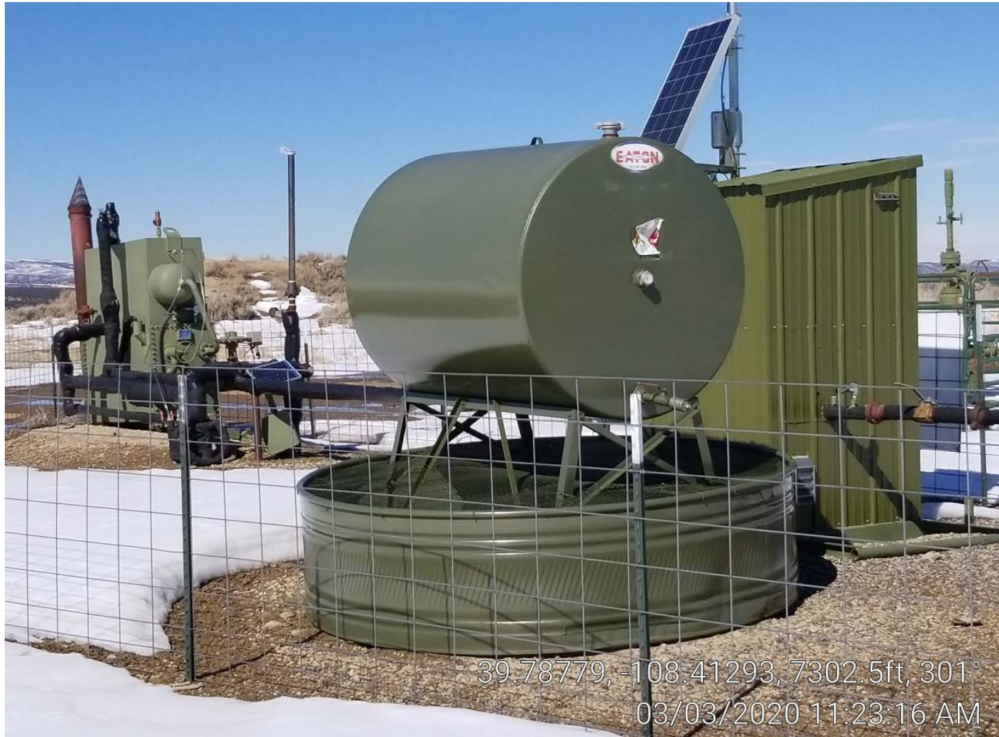
Photo 2. Separator, chemical, and meter building.
