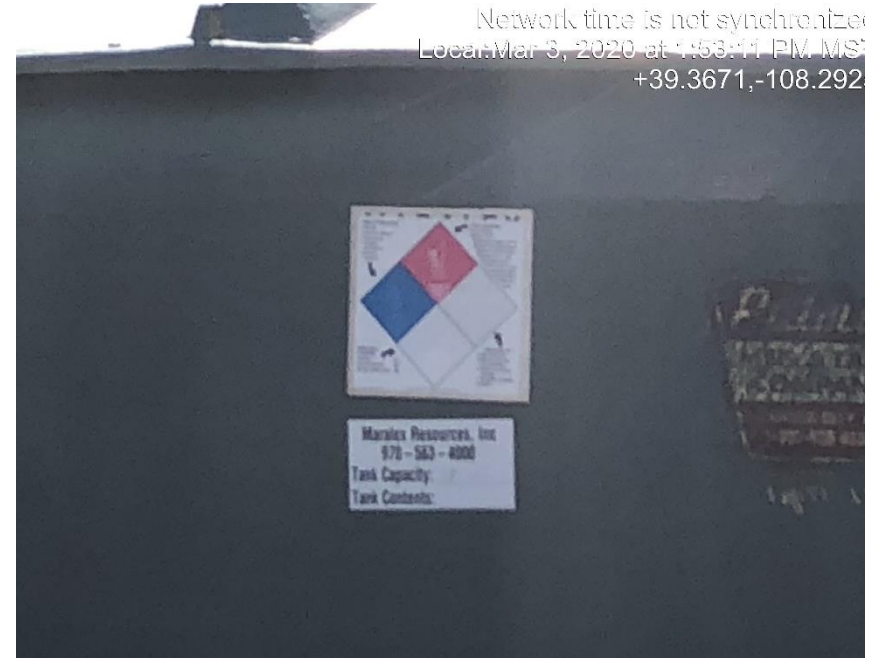
Photo #0697 Tank label weathered and not legible.
