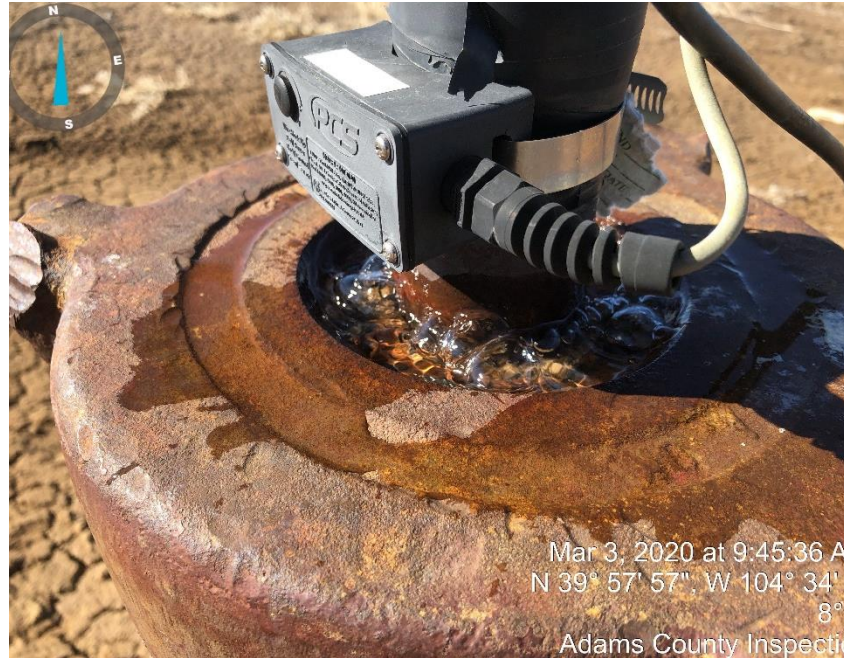
Photo #5 leak at wellhead
