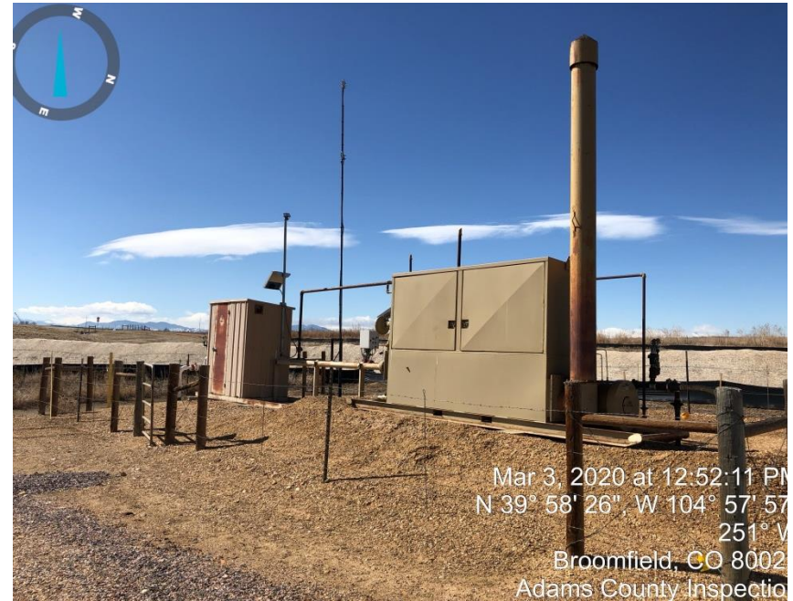
Photo#2 Separator/Gas Meter/Automation RTU
