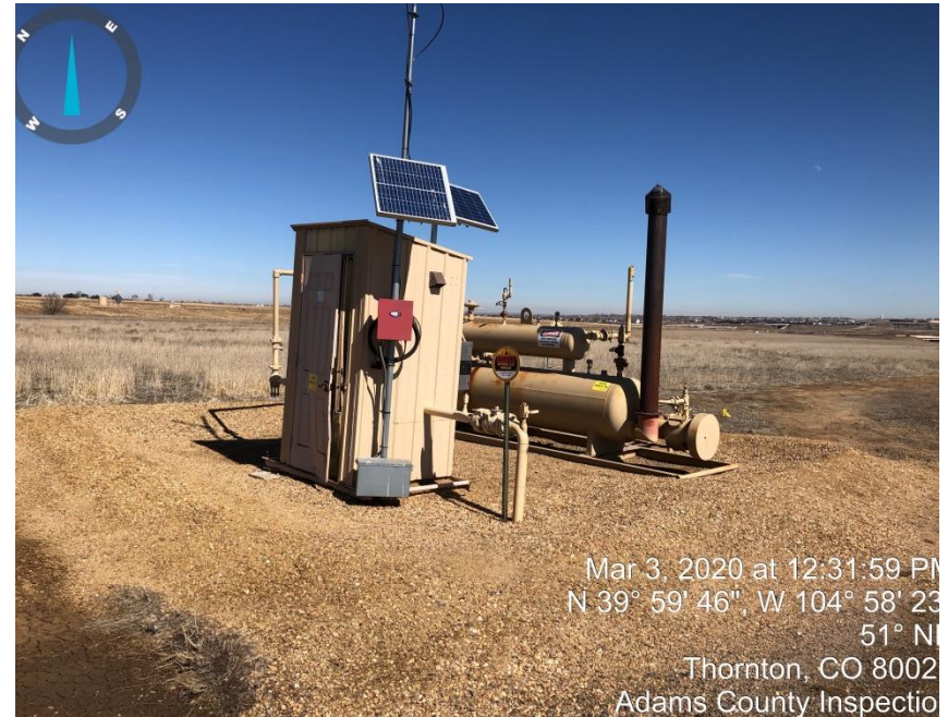
Photo#2 Separator/Gas Meter/Automation RTU
